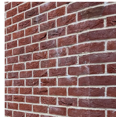
Brickwork Charnwood, Horsham Ruftrec finish Half-lap stretcher bond To match the brickwork of the Performing Arts Building at Channing School)
