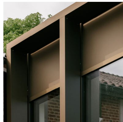
Anodised aluminium Standing seam fix Colour: Bronze (to match the aluminium of the Performing Arts Building at Channing School)
