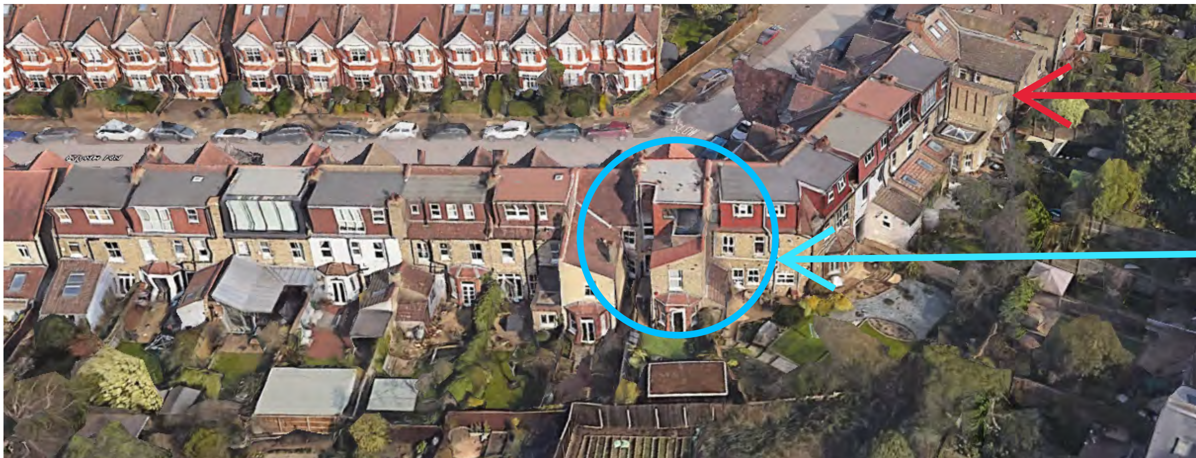
Contextual site photo showing no. 35 Clyde Road in blue
