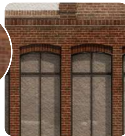
Sprung arch brick detailing and windows
