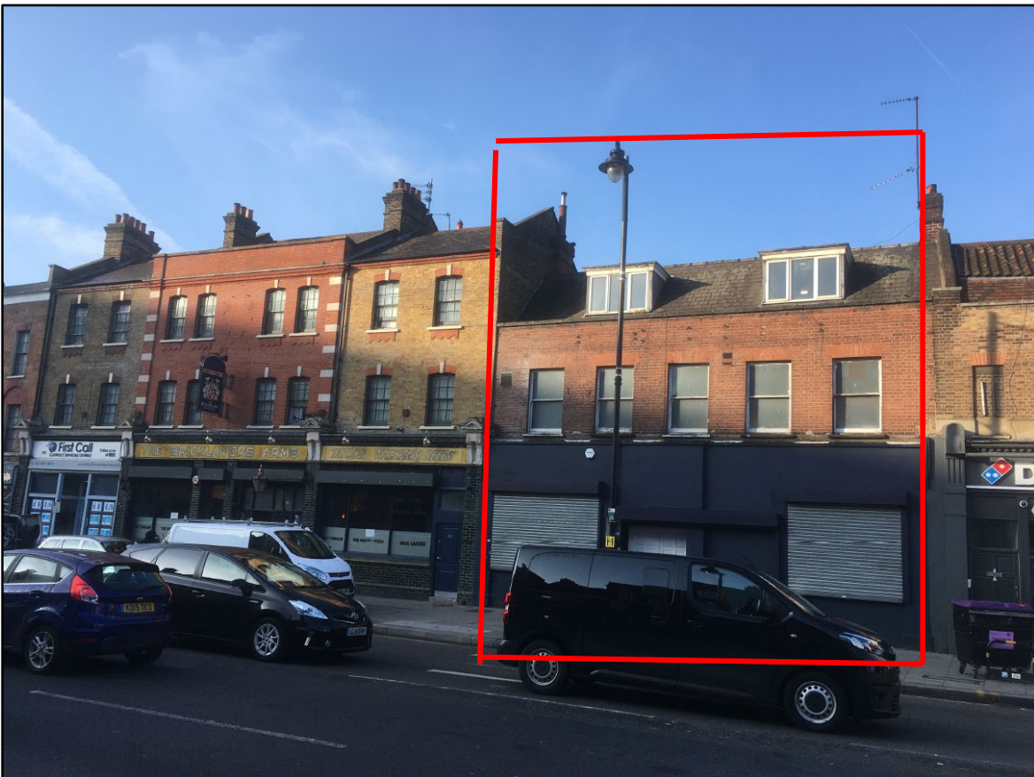
Existing High Road frontage
