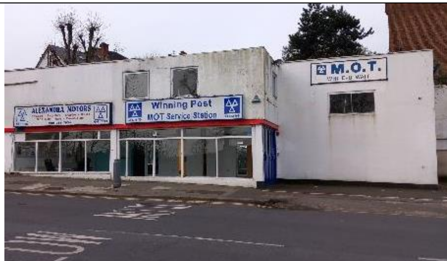
Photo 1: B1 – East elevation. B1 is a detached, brick-built commercial dwelling with a flat roof.
