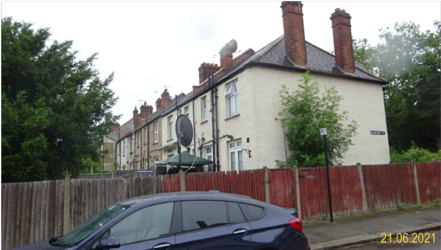
4.2 - View of the property at No.106 Downhills Park Road from Higham Road
