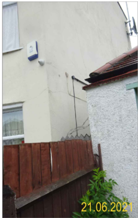
4.4 - View of the existing gap between the existing garage and the property at No.194 Higham Road
