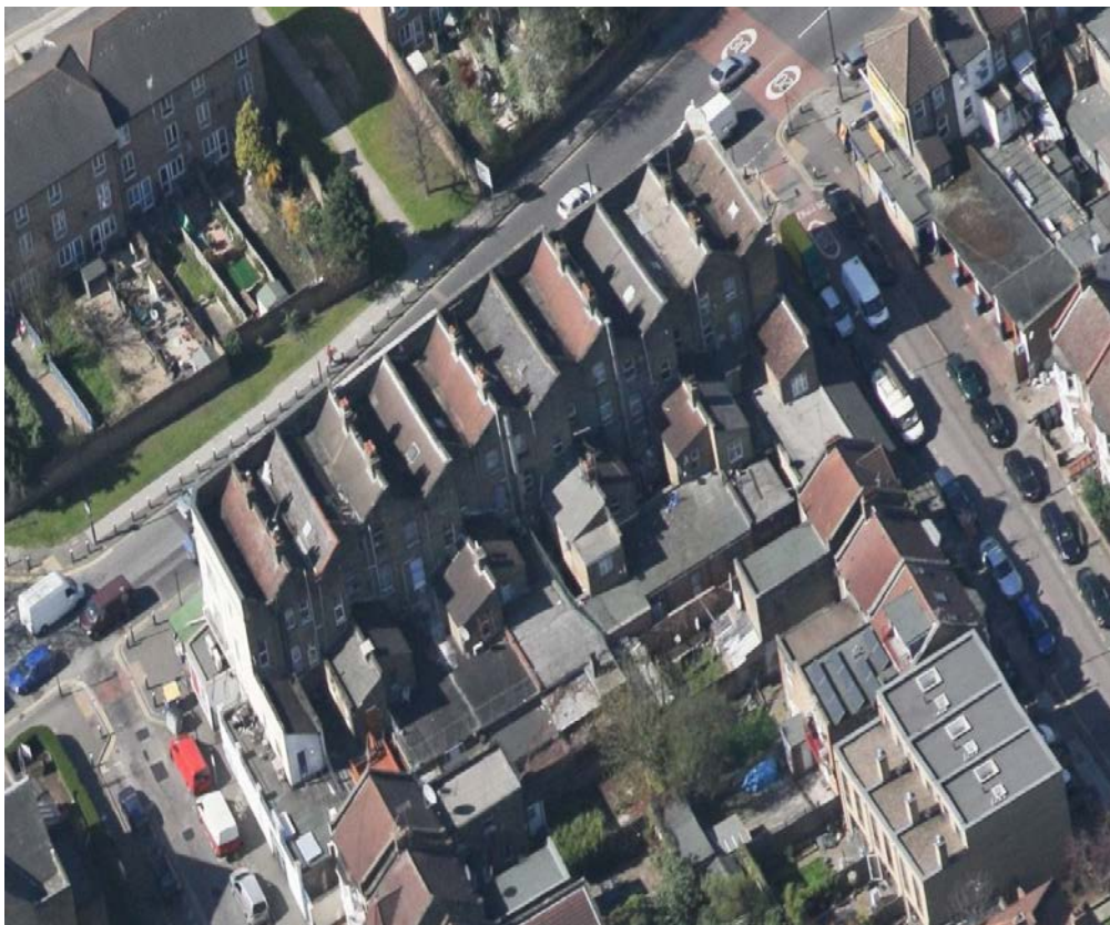
View 6 - Top view of 280 - 298 Wightman Rd. Rear Facades
