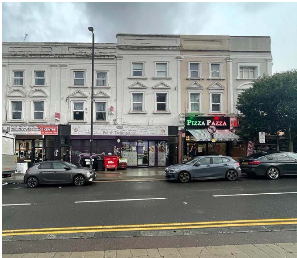
View 2 - Overlooking 288 - 280 Wightman Rd. Front Elevations
