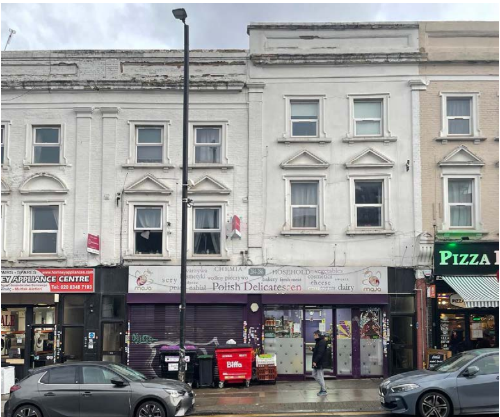
Existing Front Elevation - Photo
