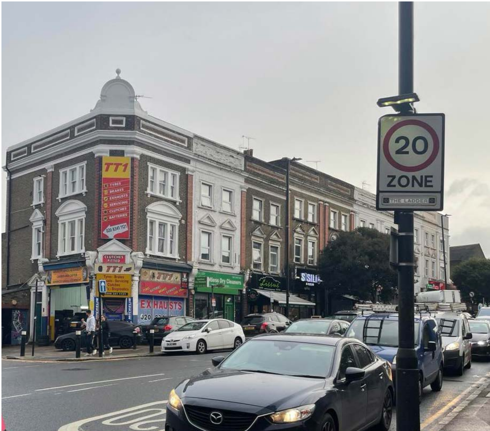
View 1 - Overlooking 298 - 280 Wightman Rd. Block of Buildings
