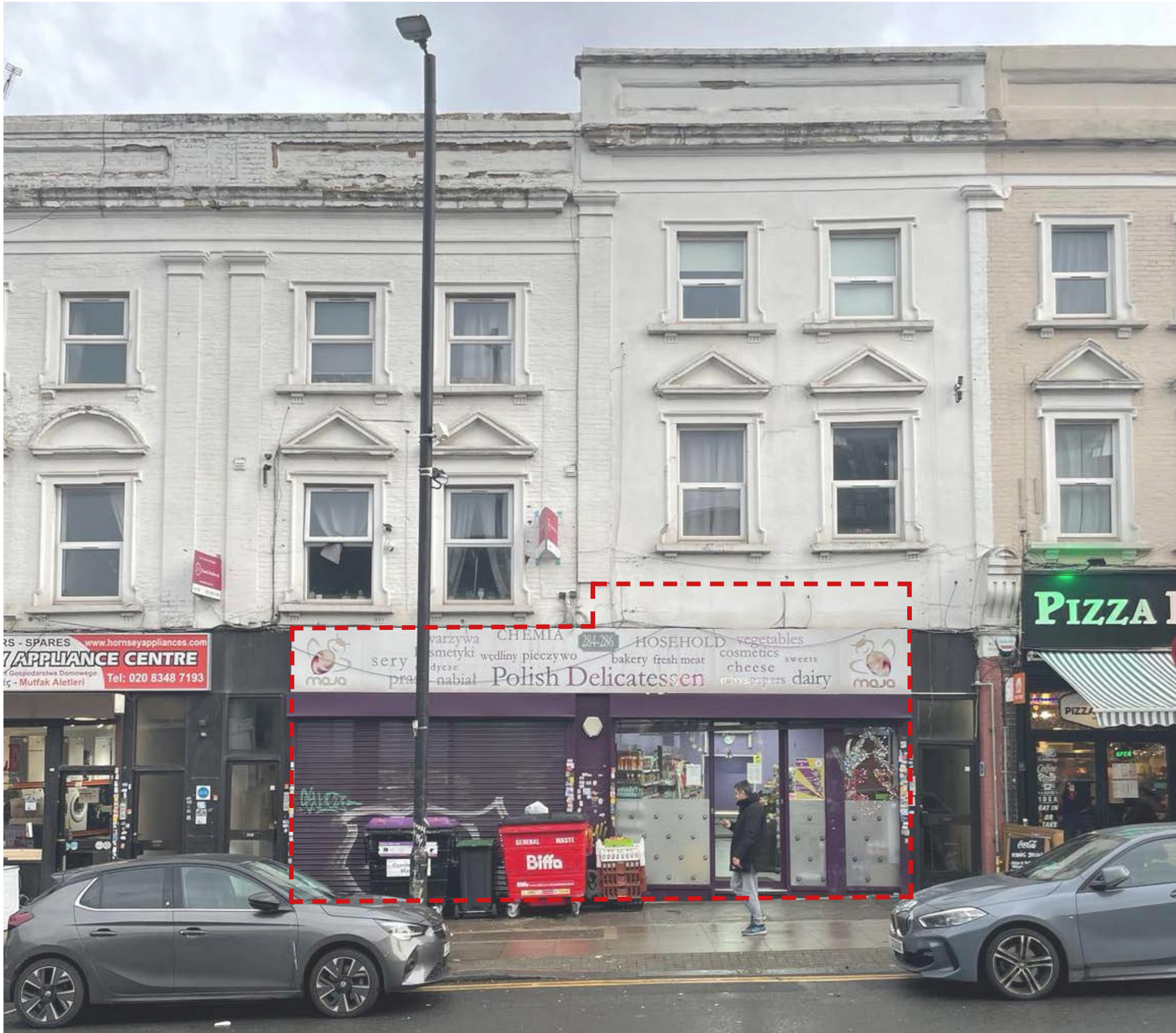
Existing Building - Wightman Road
