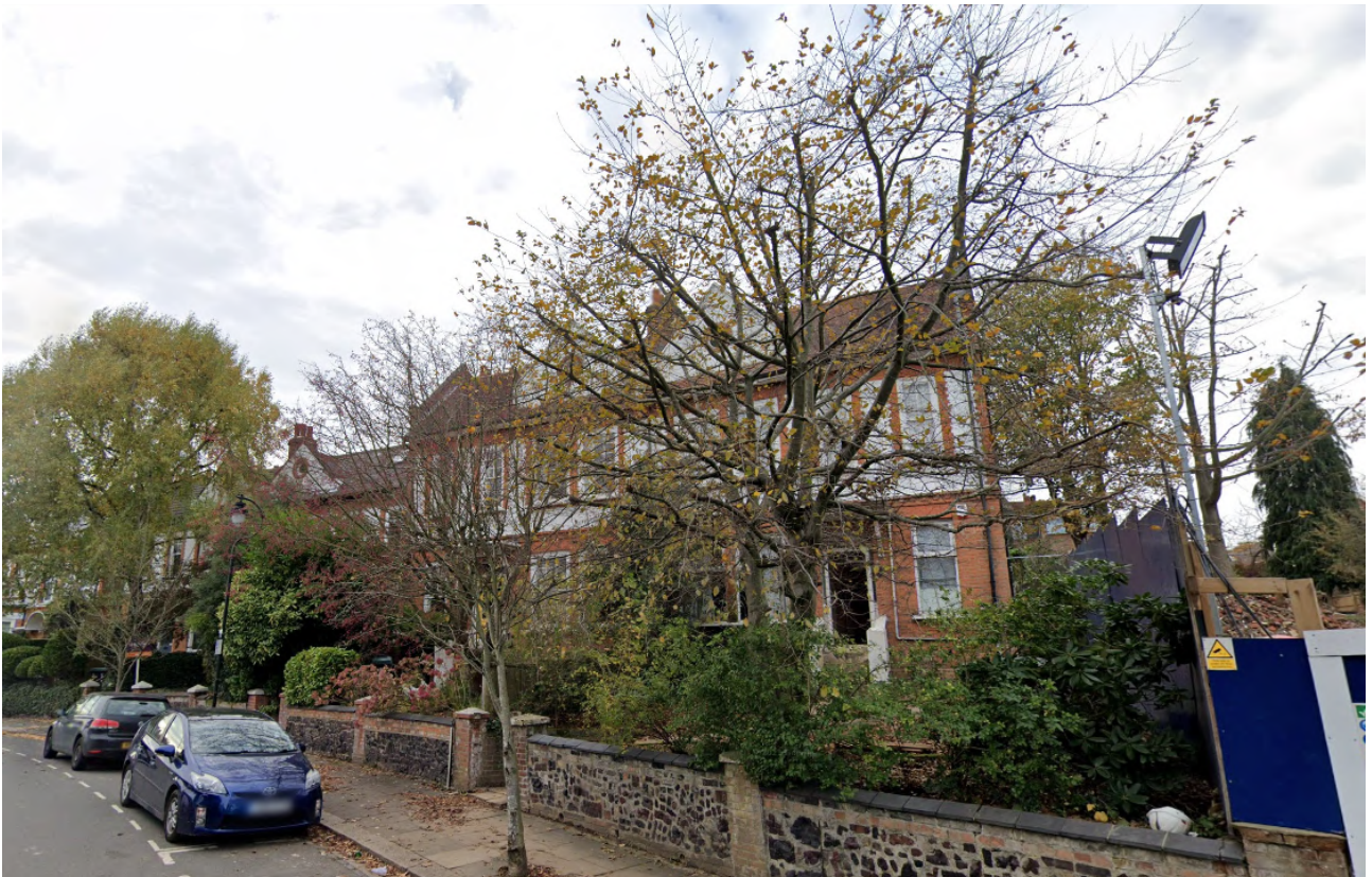
Fig.2 Street scene along Cholmeley Park, in general the works only seek to retain and enhance the front elevation, this being the prominent heritage asset in the conservation area.
