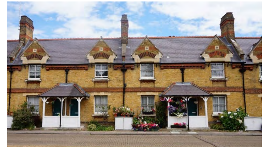
Figure 4.3. View of almshouses fronting onto gardens.
