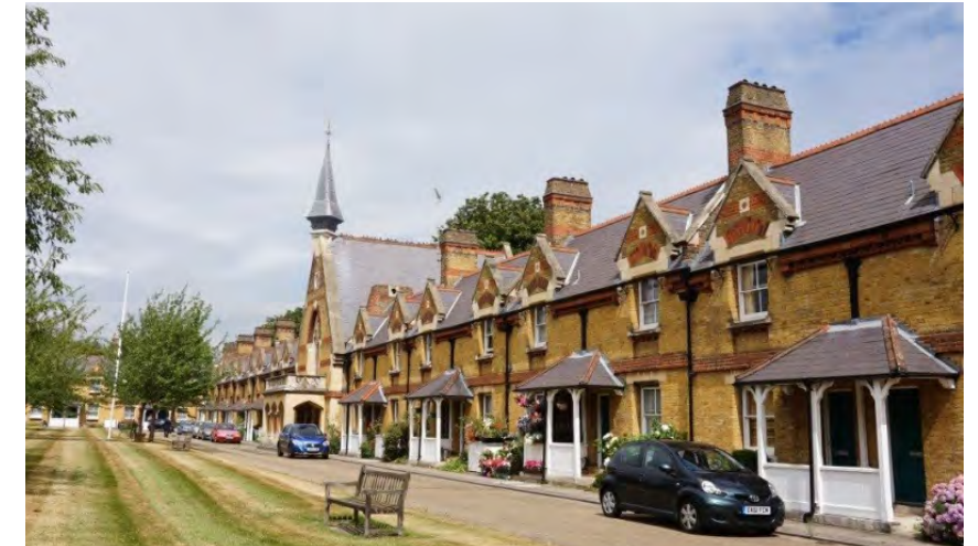
Figure 4.2. View of the Chapel and residential terraces.
