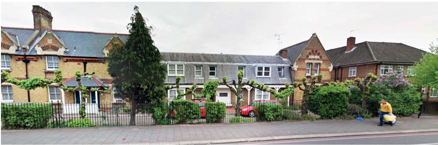
VIEW 2 - VIEW OF THE 1970'S INFILL BUILDING
