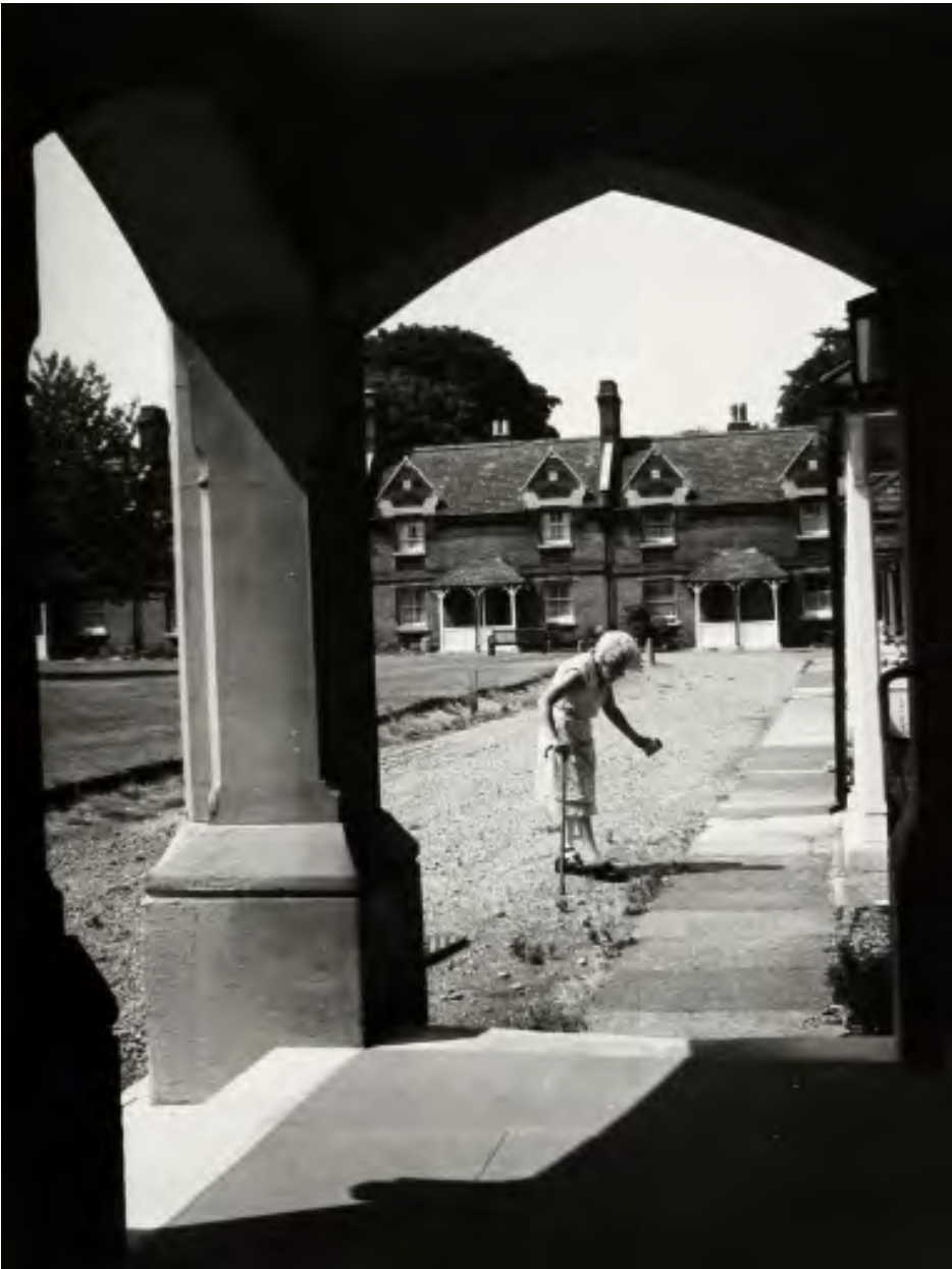
Figure 3.4. 1976 Photograph showing the Almshouses as viewed from the porch of the Chapel.
