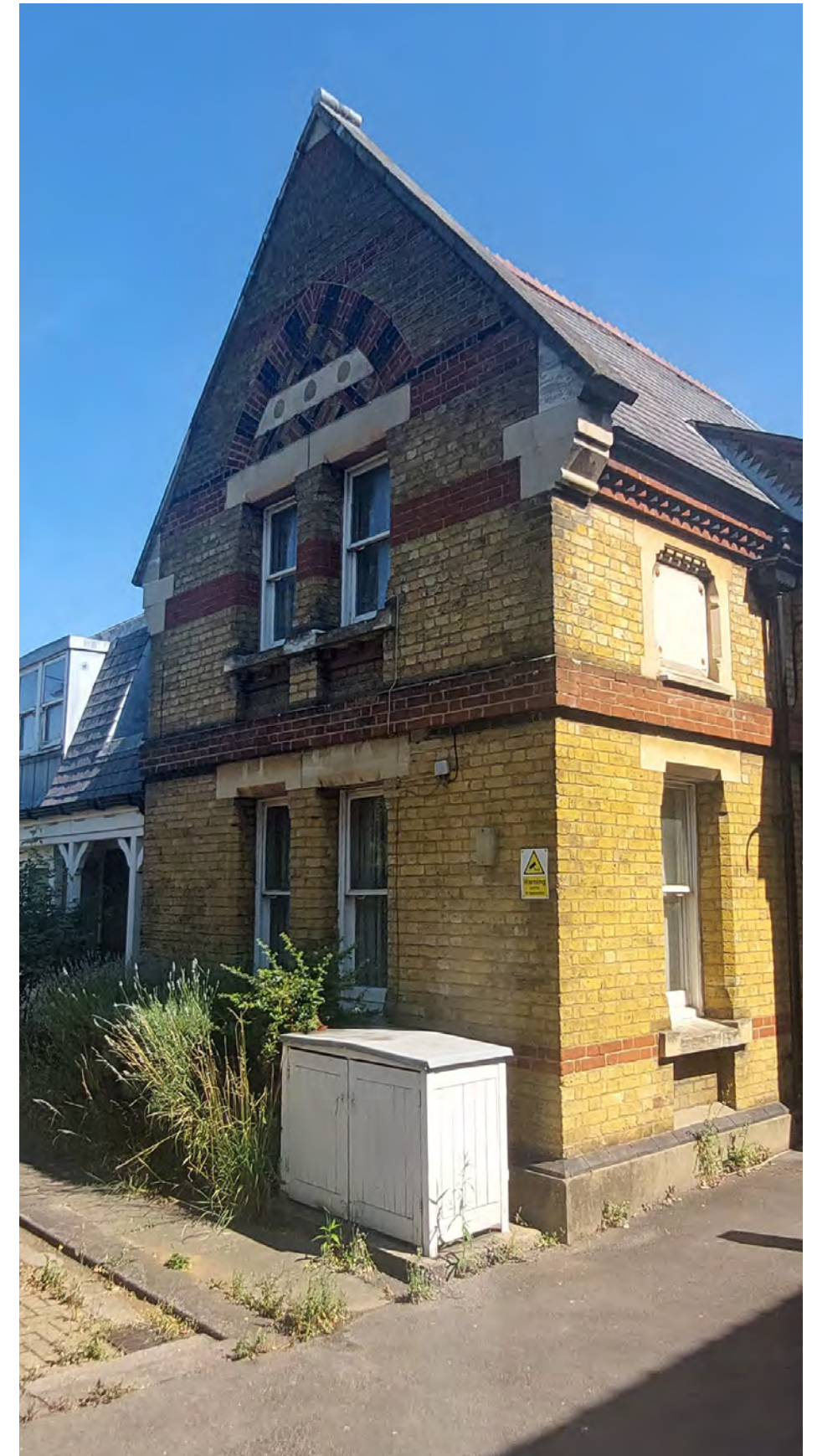
Figure 4.1. The Lodge at the entrance to the site.
