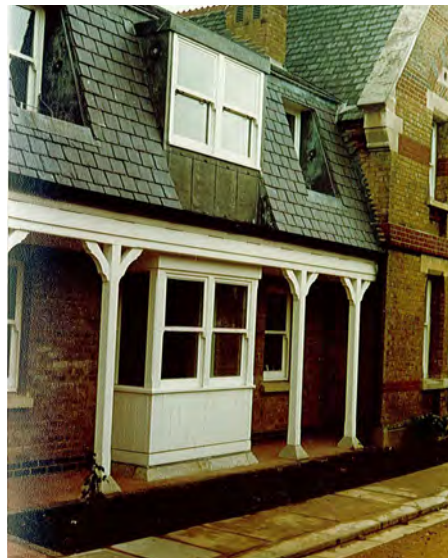
Figure 3.6. New infill between the Matron's Lodge and main Almshouse blocks designed by Berry Webber & Partners, architects and built 1978-1981. © Drapers' Company Archives.
