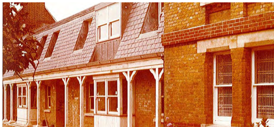
Figure 3.7. New infill between the Matron's Lodge and main Almshouse blocks designed by Berry Webber & Partners, architects and built 1978-1981. © Drapers' Company Archives.
