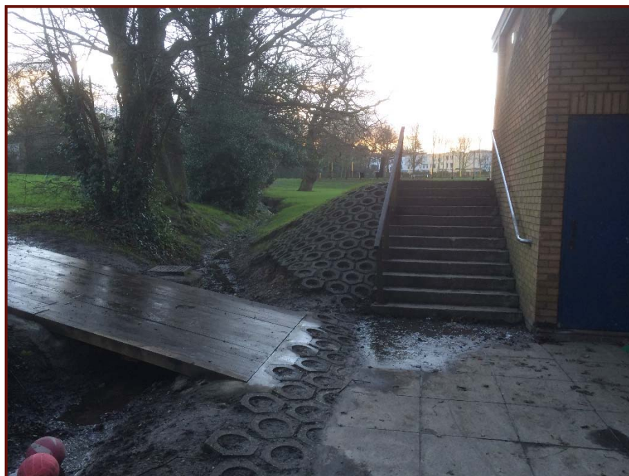
Steps up to higher-lying area adjacent to sports hall; drainage ditch on left (looking SE)
