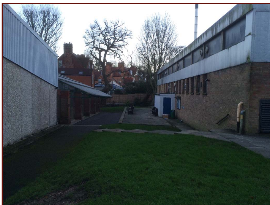
View along side of swimming pool boundary with games courts on left (looking NE)
