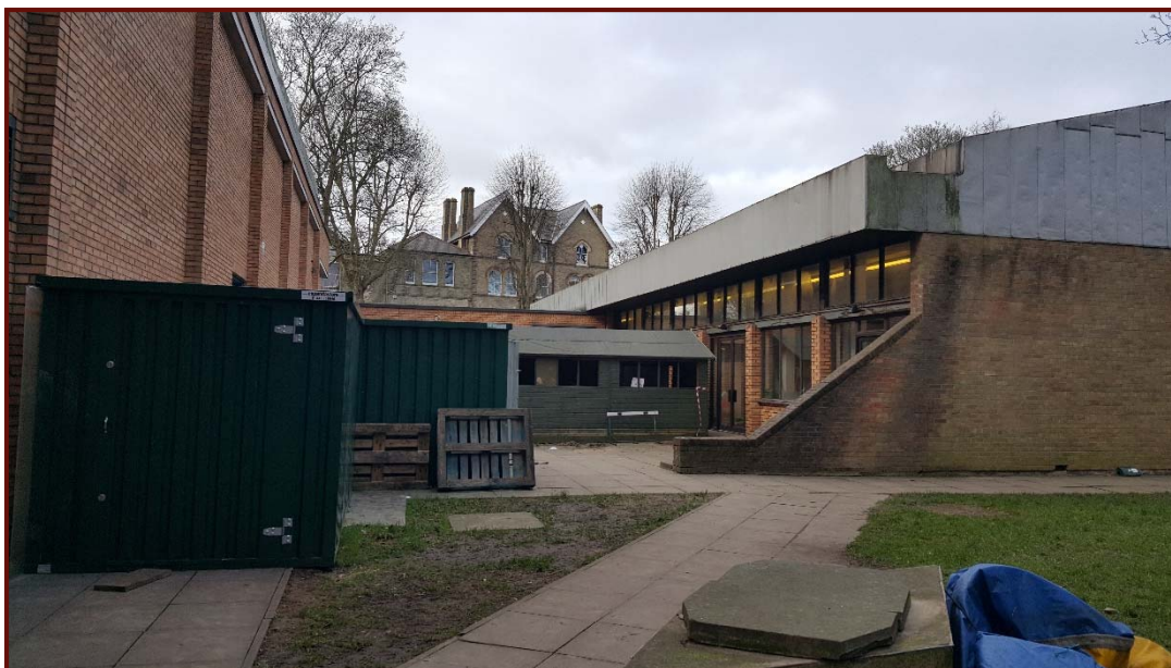
General view of 'courtyard' area (looking SW)
