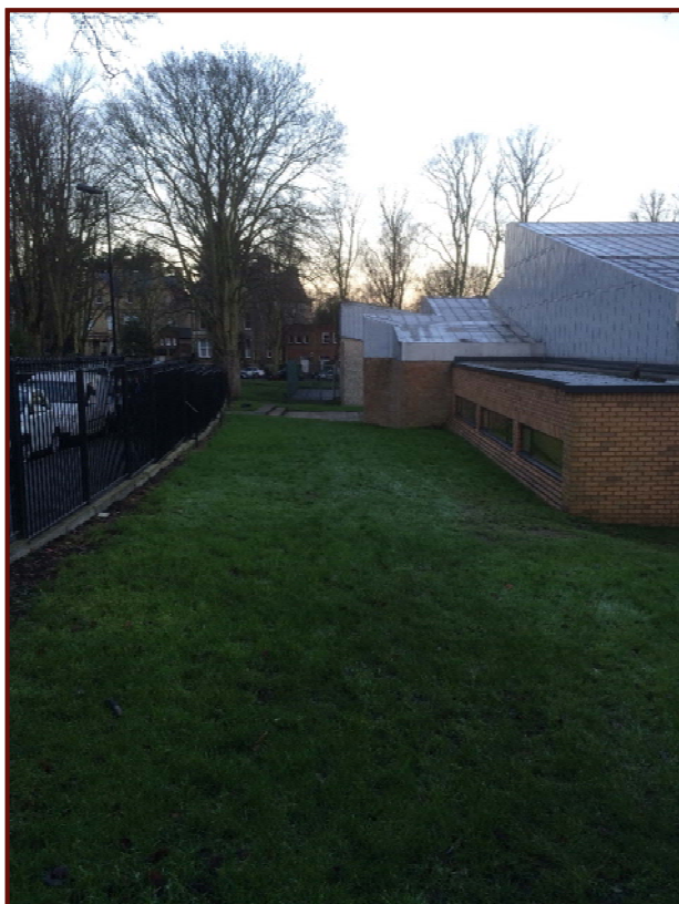
Bishopswood Road boundary (looking NW)
