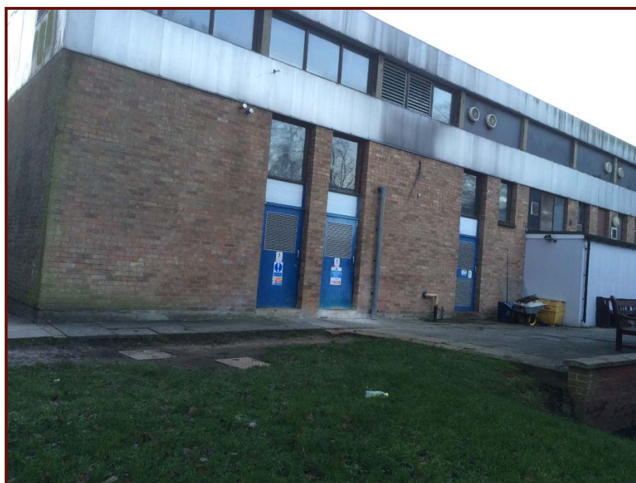
Swimming pool building showing plant rooms (looking S)
