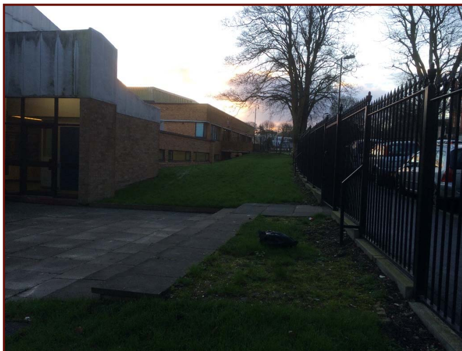
View along Bishopswood Road boundary (looking SE)
