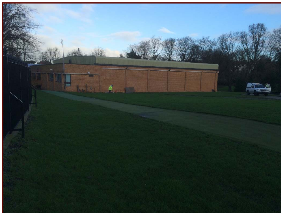
General view of NE elevation of sports centre (looking NW)
