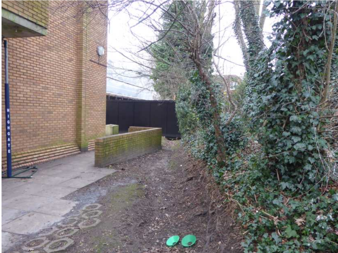
Figure 2.4: Existing ditch to the rear of the existing Mallinson Sports Centre requiring clearance and improvement.
