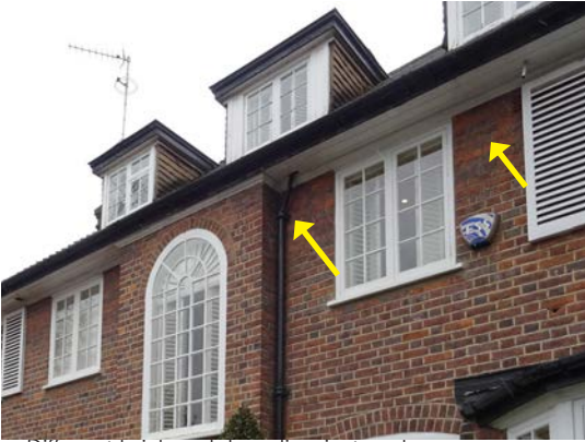
e. Different brickwork banding just under eaves.
