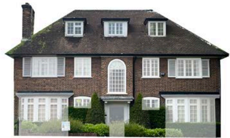
Windows & doors demolition
