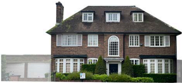
Side extensions demolition
