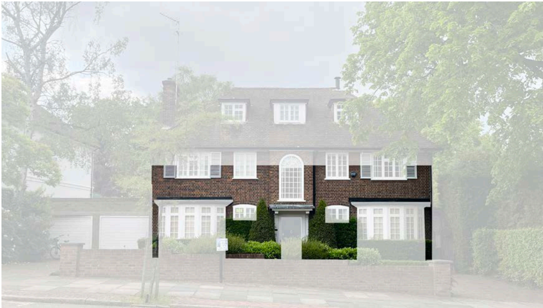
Facade to be retained - after demolition
