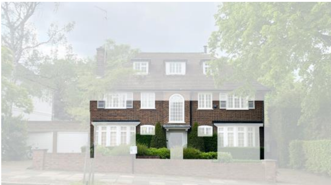
Facade to be retained - after demolition, image by MWA
