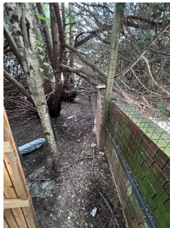
Figure 2 – Retained Garden and Trees Behind Wall
