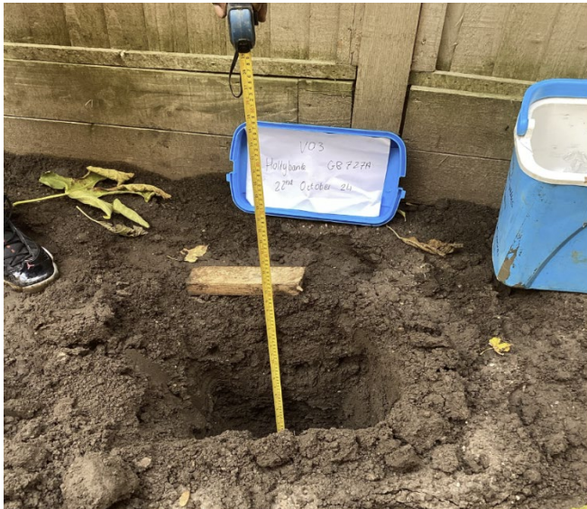
Photo 5: V03 Inspection Pit
