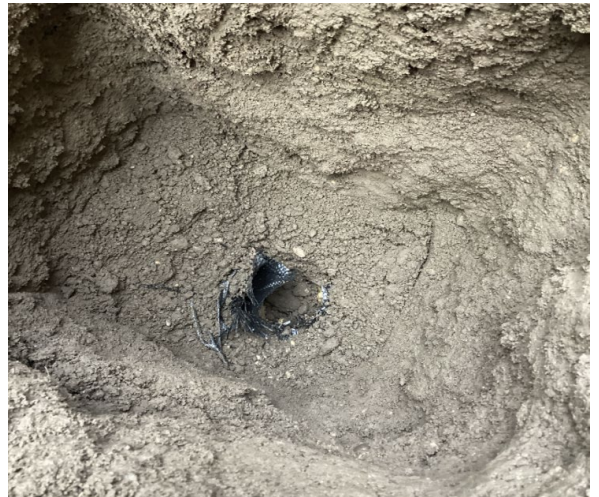
Photo 2: V01 inspection Pit
