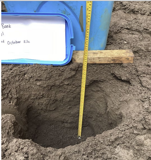
Photo 1: V01 Inspection Pit
