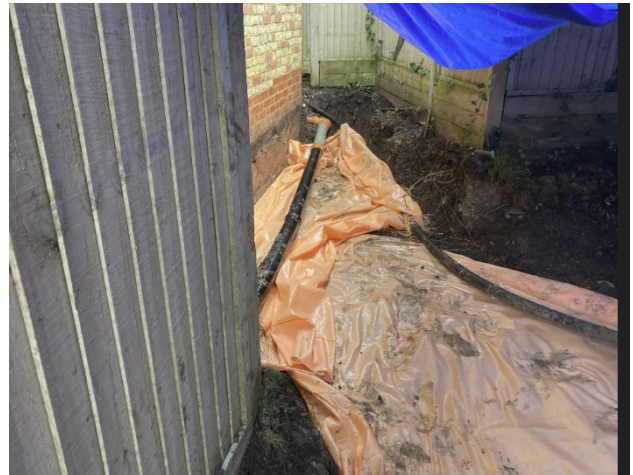
Photo 10: Membrane verification
