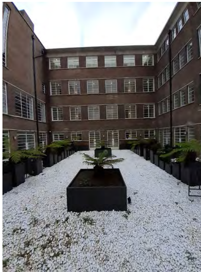
41 South elevation of Link Block, now Hotel corridor and rooms
