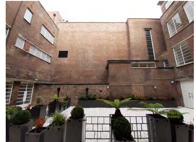
42 Service Court elevation looking north
