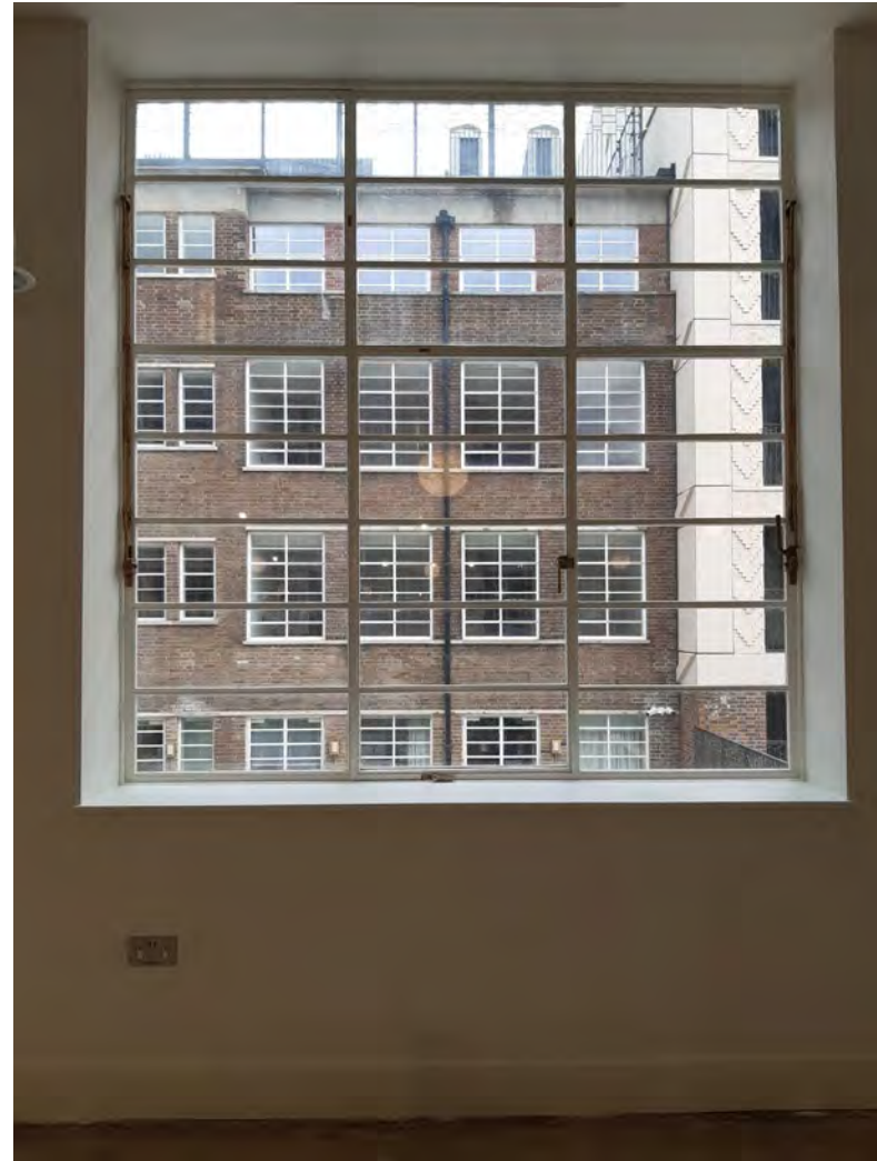
80C G.27 original windows to co-working space
