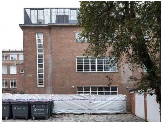
35 Rear (east) elevation of Assembly Hall Block
