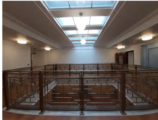
142 S.32 Open lightwell looking south
