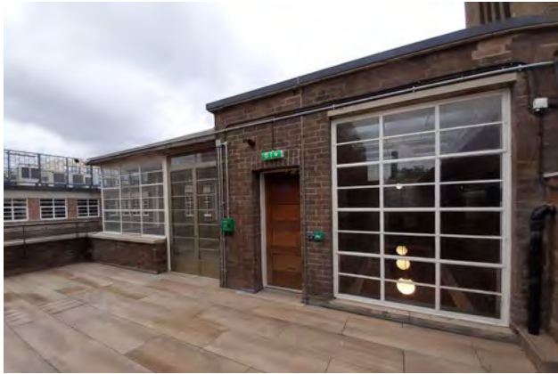
44 Flat roof over Assembly Hall Block
