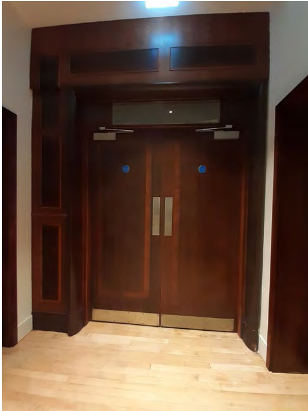
98 G.64 Exit Lobby
