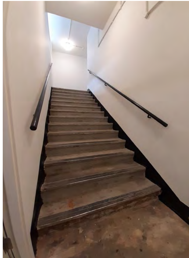
157 ST.10 basement to ground
