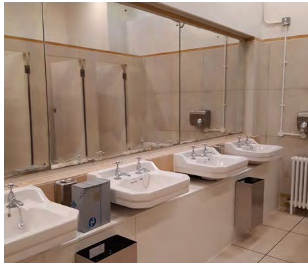
92A G.54 Ladies Lavatory looking east
