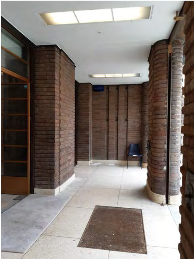
89A G.49 Vestibule looking south
