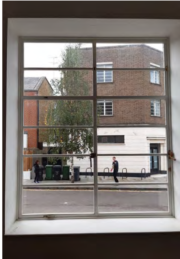
81C G.38 F&B Restaurant windows (original)
