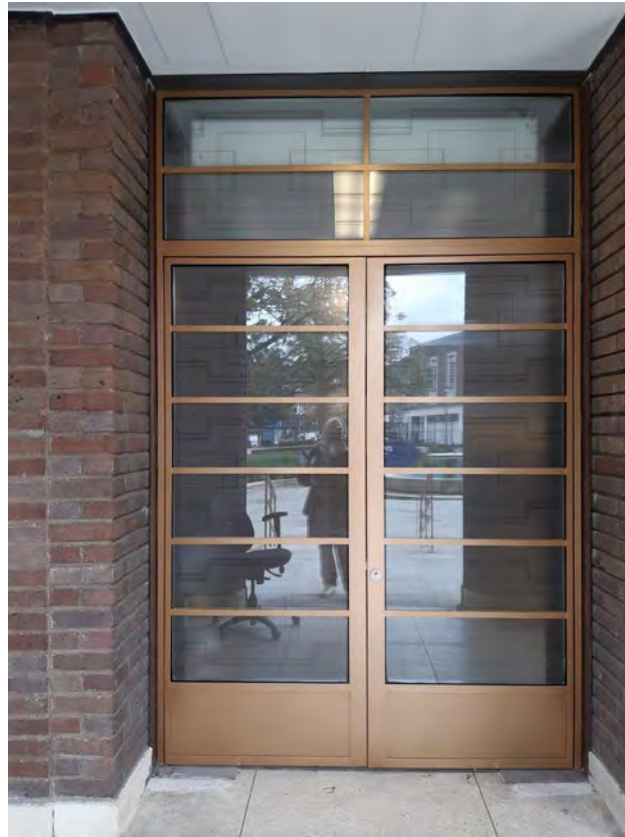
89B G.49 Vestibule, new entrance doors
