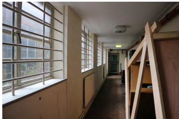
53C LG.20 Basement, corridor in Link Block (2017)
