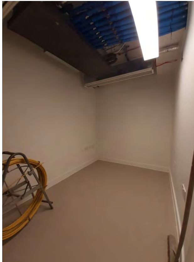
55 LG.21b Maintenance Store
