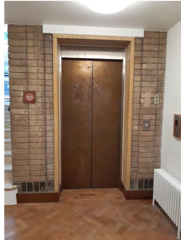
50B lift doors
