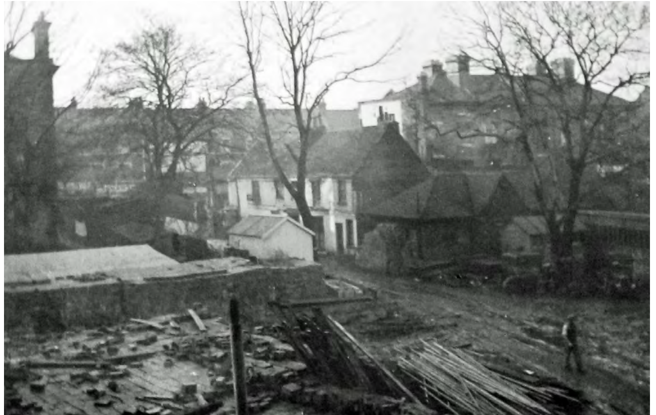
6C Forecourt area, 1934 (Haringey Archives)
