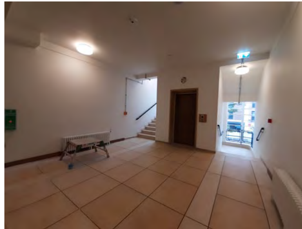
78 G.17 Ground Floor Landing - 1
