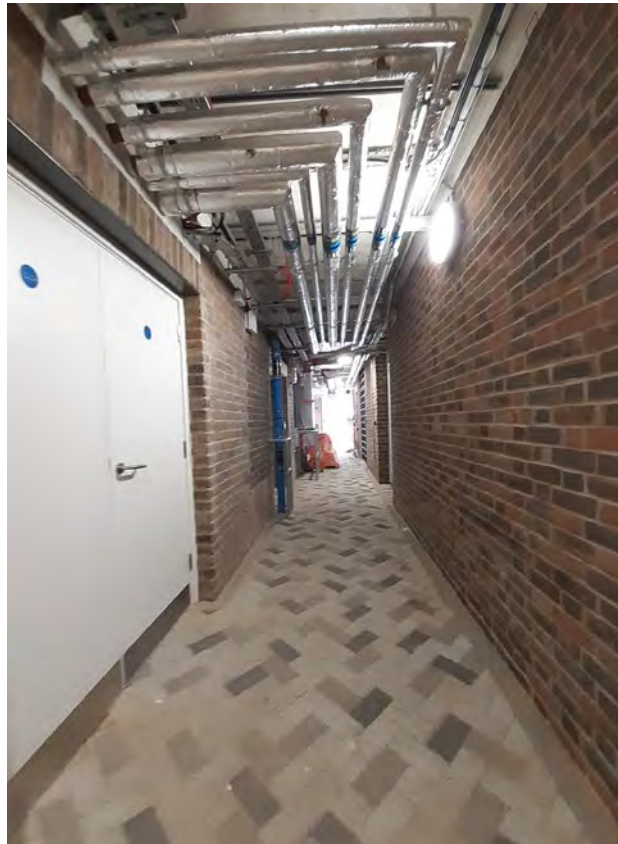
66 LG.45f New covered corridor near Plant and Refuse Store
