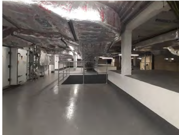
65 LG.43 Plant Room beneath Assembly Hall 1
