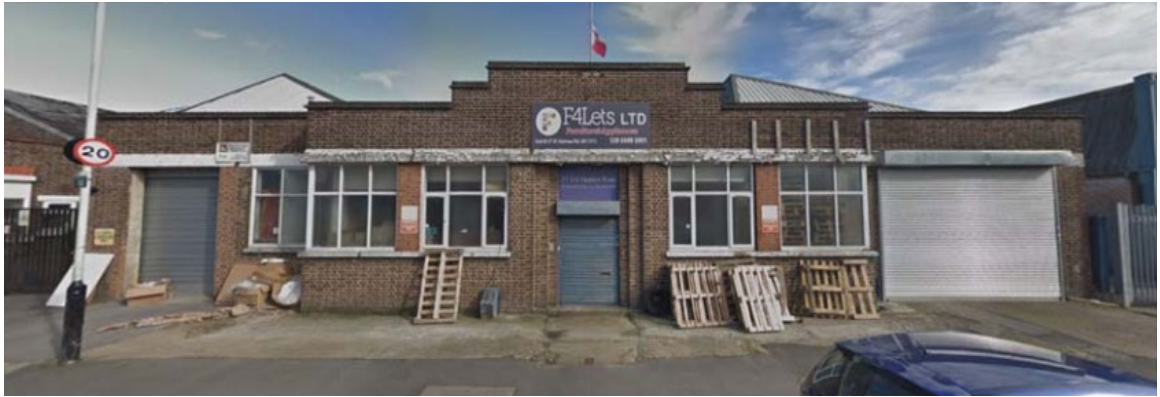
Photograph of pre-existing building
