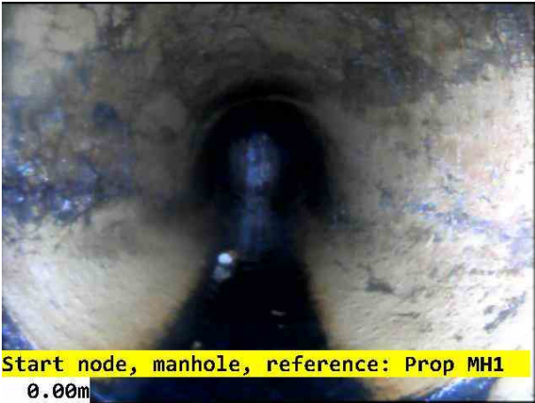
Prop MH2X_04448ee3-2b99-48af-a5f7-3f29f4c71ea5_20210608_22 3311_452.jpg, 00:00:00, 0.00 m Start node, manhole, reference: Prop MH1, Start
