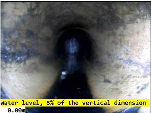
Prop MH2X_b0971c87-47ae-4348-8f72-602ae474ae10_20210608_ 223345_105.jpg, 00:08:25, 0.00 m Water level, 5% of the vertical dimension, live flowing water
