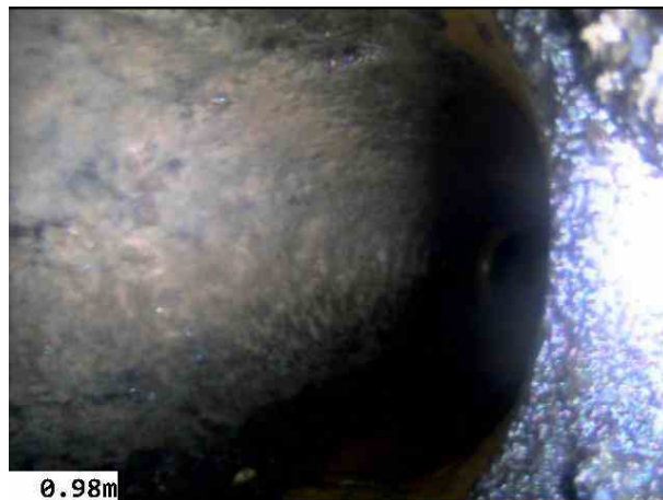
Prop MH2X_b69b6607-2d40-46c7-aa44-2af71f9207bb_20210608_2 23918_244.jpg, 00:01:15, 0.98 m General photograph taken at this point, Poss backdrop in pipe
