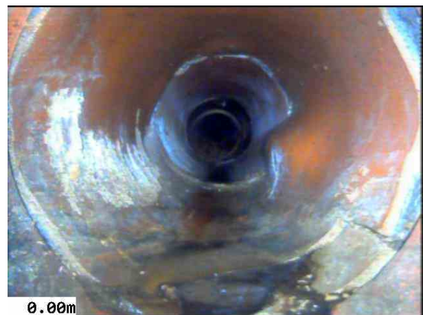
Garden 1X_d8896931-0468-4495-b516-d9d9ac0b8949_20210608_212 912_178.jpg, 00:00:00, 0.00 m Start node, manhole, reference: Prop MH1, Start
