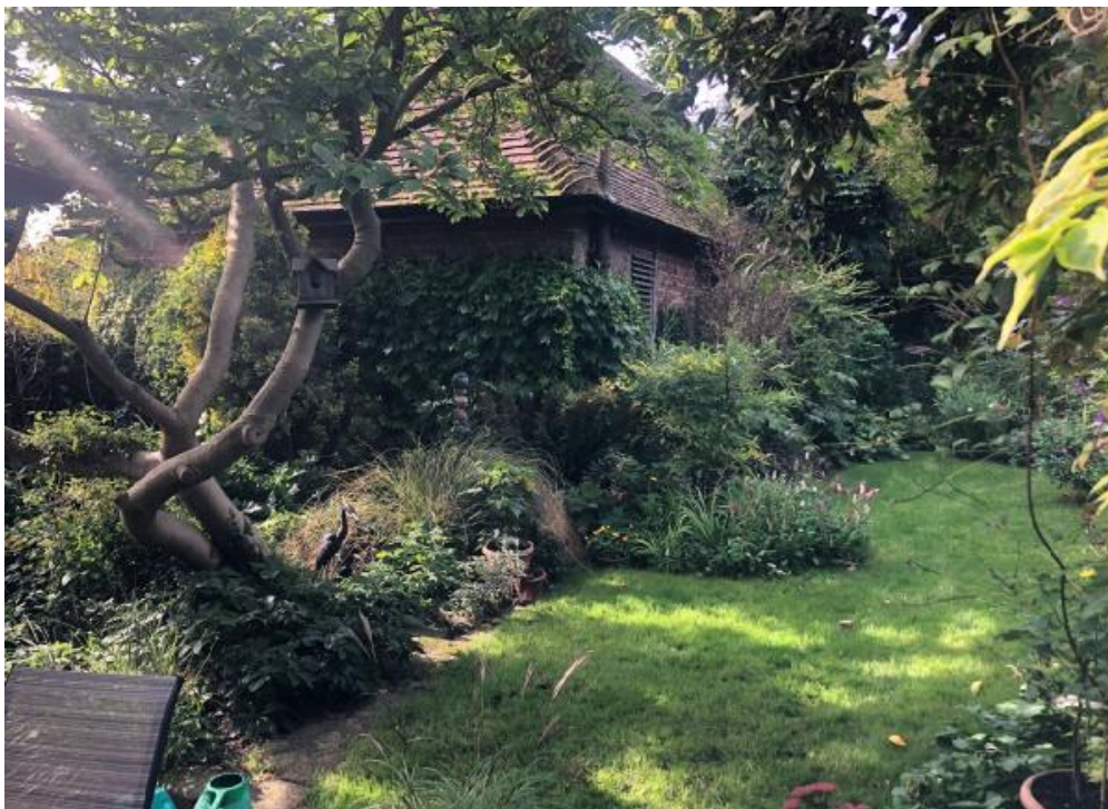
Figure 12: Existing rear elevation to the pavillion as seen from garden of No No.37 Cascade Avenue
