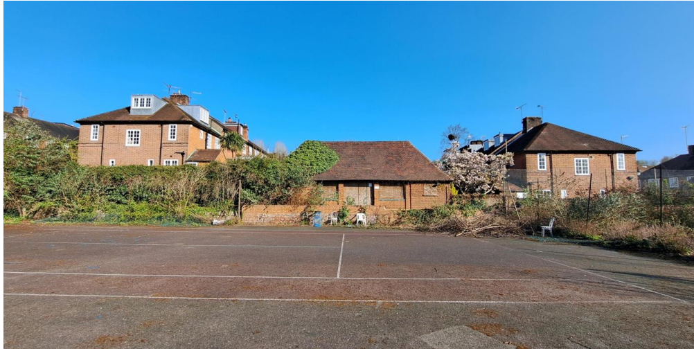
Figure 3: Current conditions of courts and pavilion building
