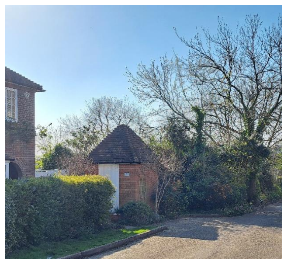
Figure 6: Outbuilding on The Chine. The pavement lies beneath the currently overgrown hedge.
