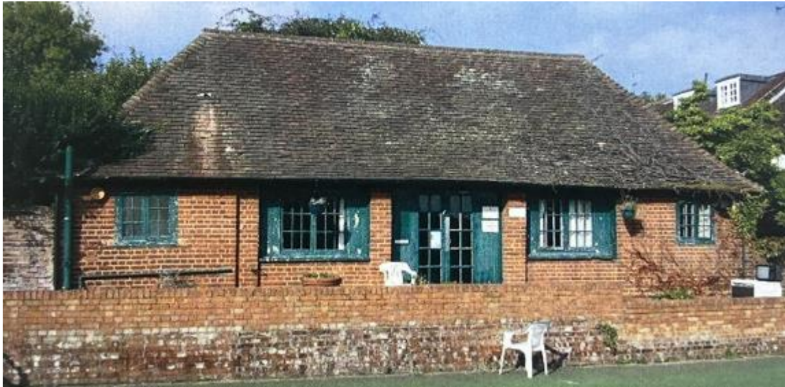
Fig. 17 The Grove Lawn Tennis Club clubhouse built by the Collins family in 1912. As it was when the club operated
