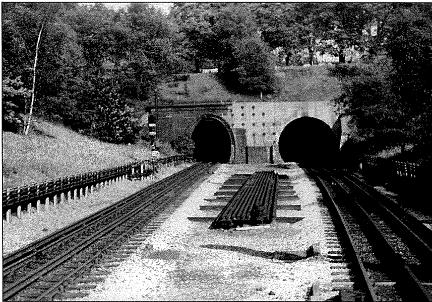
Highgate Tunnels – North End, June 1945
