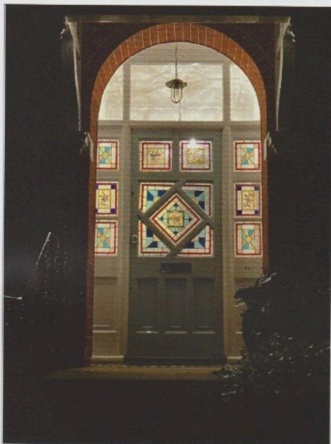
Fig. 11 Coloured glass in the front door and side panels of a Collins house in Mountview Road
