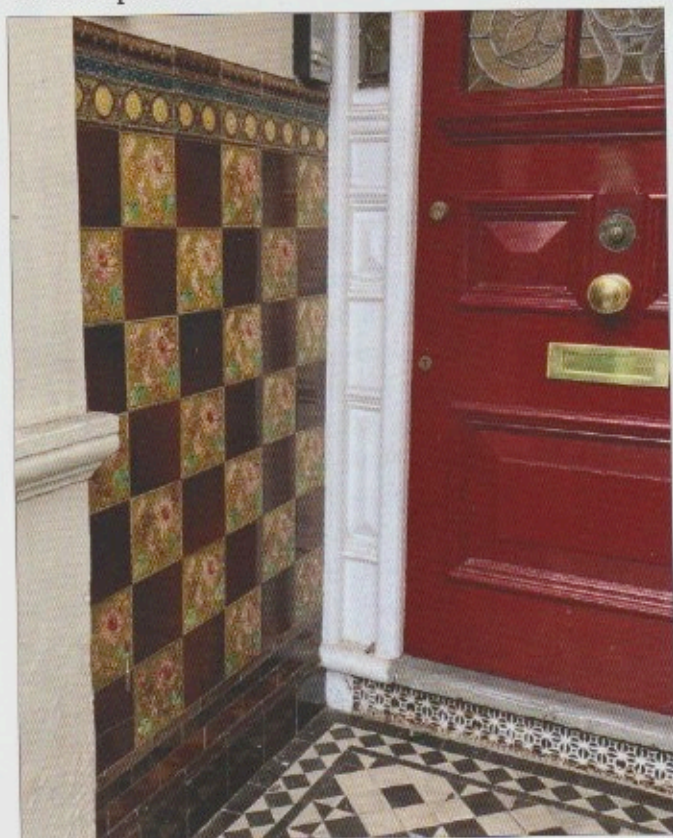
Fig. 9 Porch with dado height wall tiles on a Farrer house in Weston Park. Note the black and white floor tiles in the porch and the panelled door with coloured glass.
