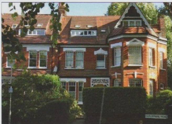
Fig. 1 Collins: Houses in Haslemere Road built in red brick and tiles with fretted bargeboards and chinoiserie porch details.
