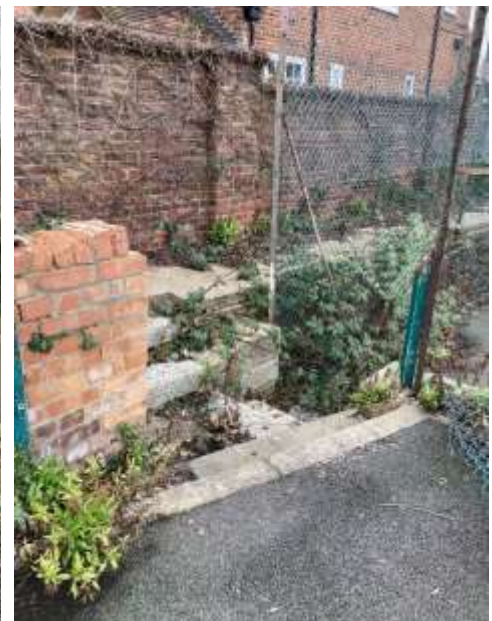
Stairs between upper and lower courts
