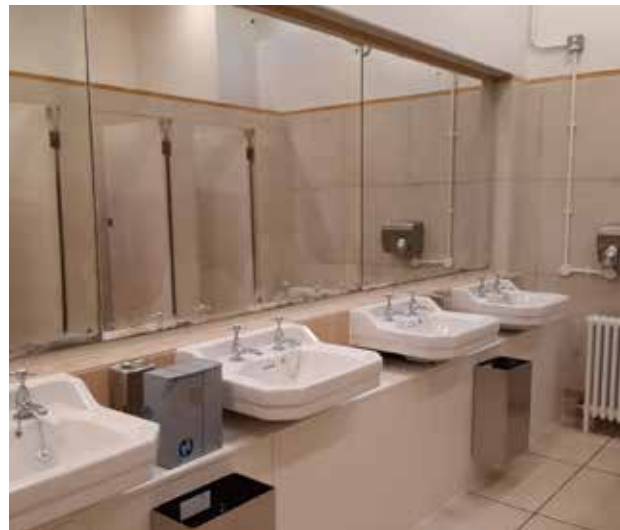
92A G.54 Ladies Lavatory looking east
