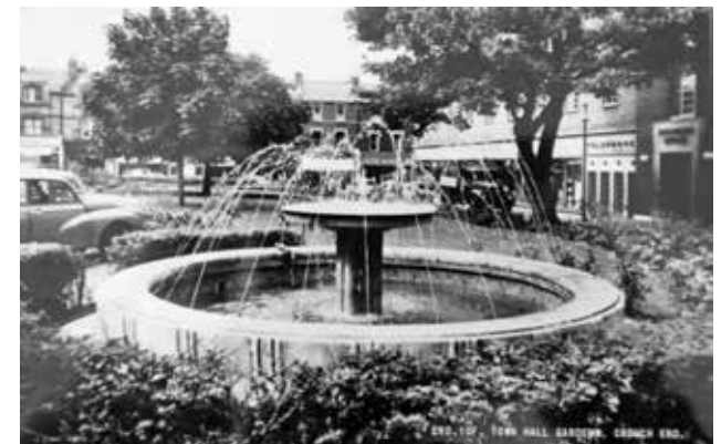
22F Forecourt and fountain, c. 1960s (Haringey Archives)
