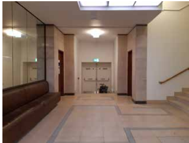
93C G.52 Corridor looking north
