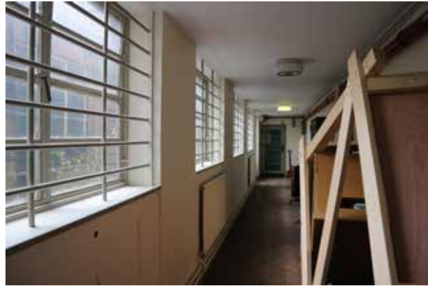
53C LG.20 Basement, corridor in Link Block (2017)
