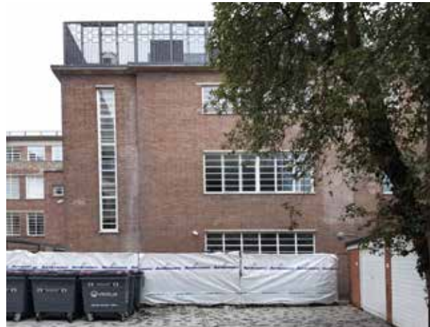
35 Rear (east) elevation of Assembly Hall Block
