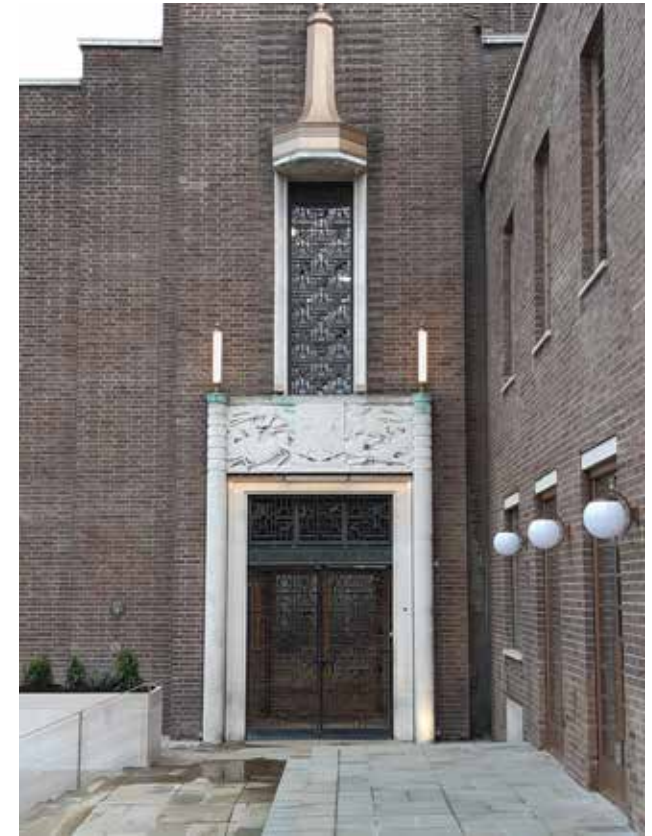
32 Carved stone doorpiece to the Administrative Entrance
