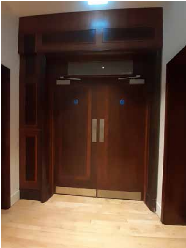
98 G.64 Exit Lobby
