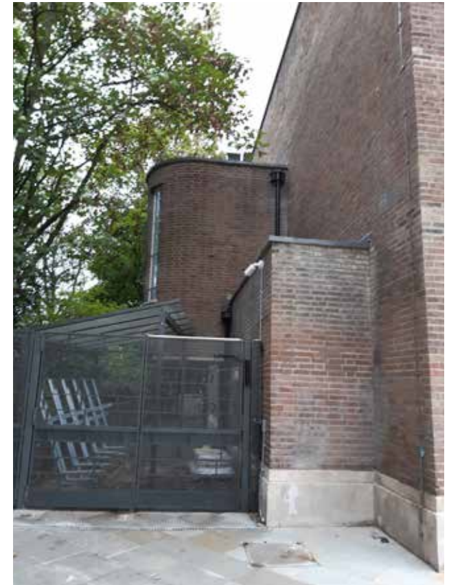
34 North elevation of the Assembly Hall Block, cantilevered stair
