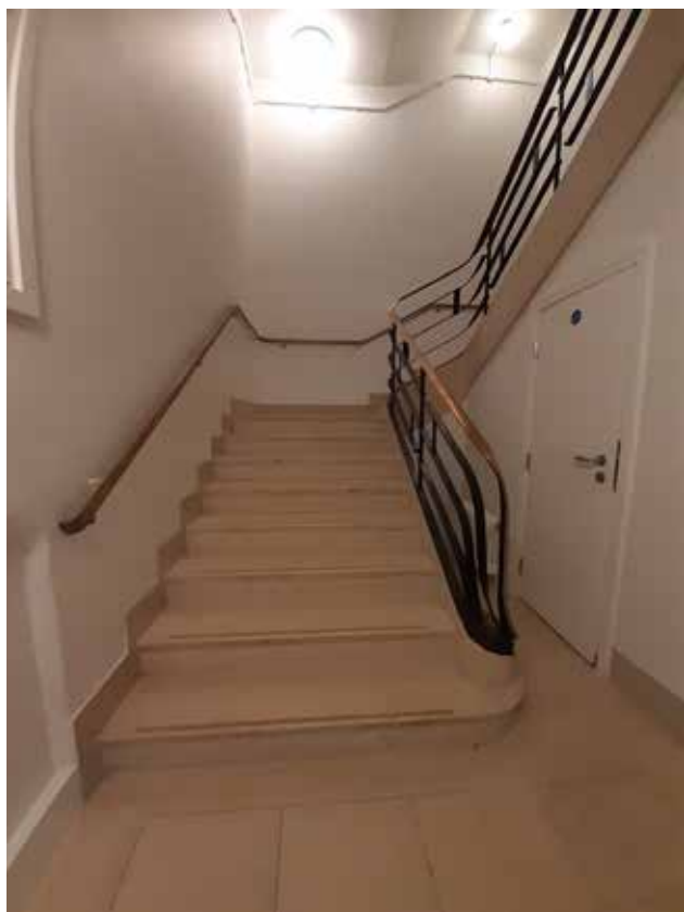
150 ST.01 view at lower ground
