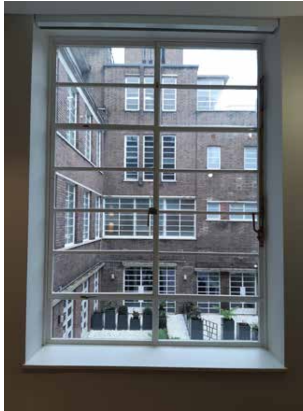
72A G.4 Original windows to corridor similar to these
