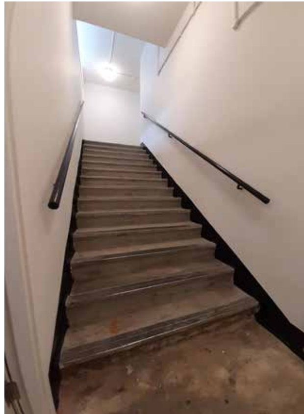
157 ST.10 basement to ground
