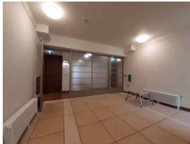
78A G.17 Ground Floor Landing -2
