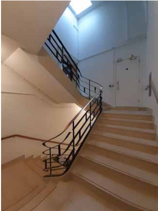
150C ST.02 second floor stair extension to roof
