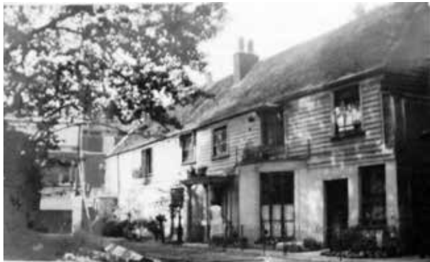
6B Cottages present on site in 1934 (Haringey Archives)
