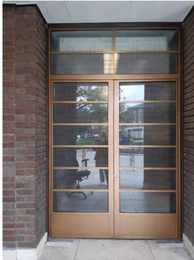
89B G.49 Vestibule, new entrance doors
