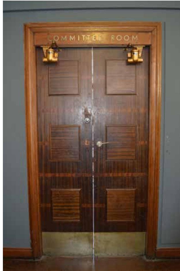
121B First Floor, Committee Room doors, F.49 (2017)
