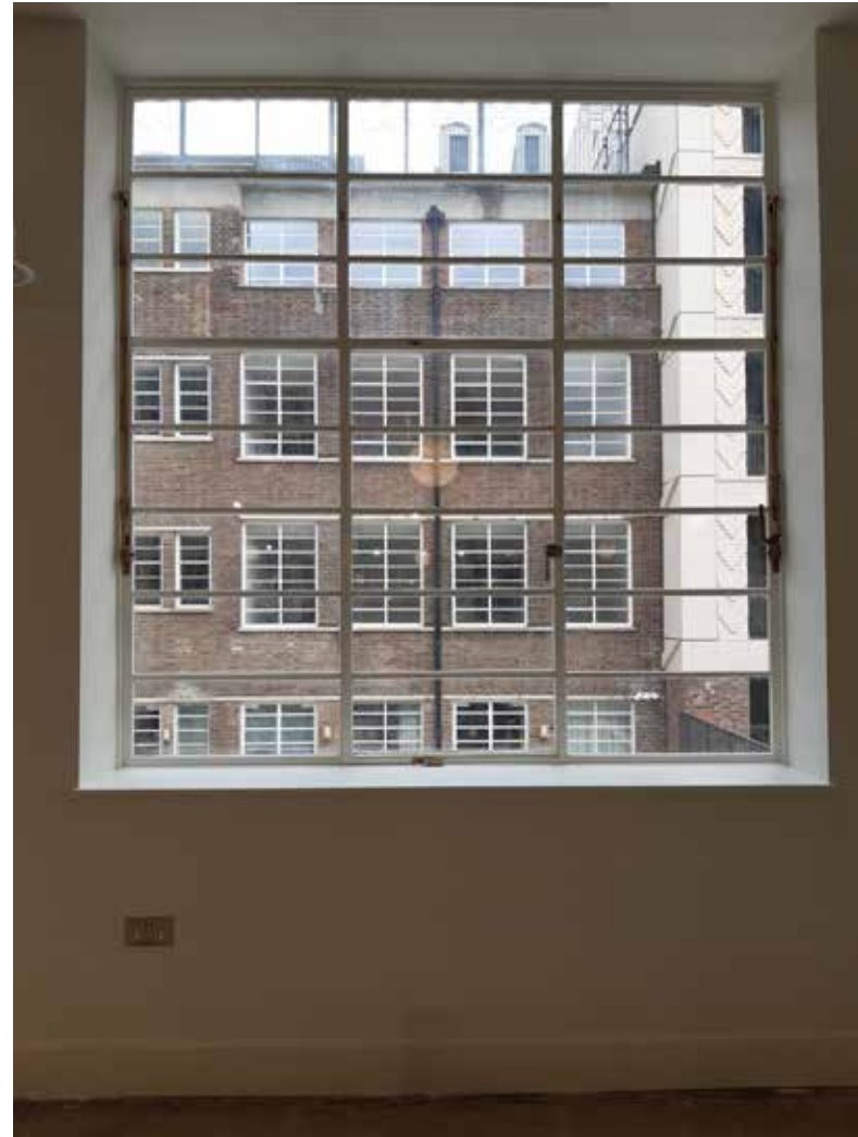
80C G.27 original windows to co-working space
