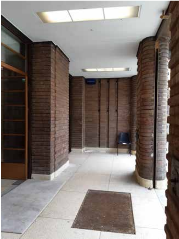
89A G.49 Vestibule looking south
