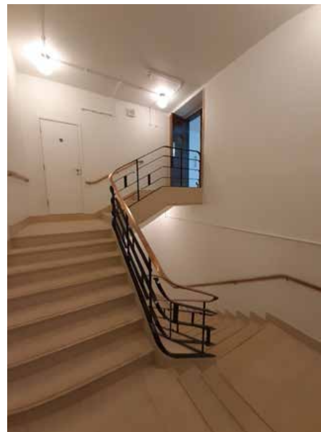
150B ST.01 view at second floor
