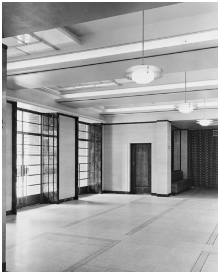
13A Assembly Hall foyer, c. 1935 (RIBA)
