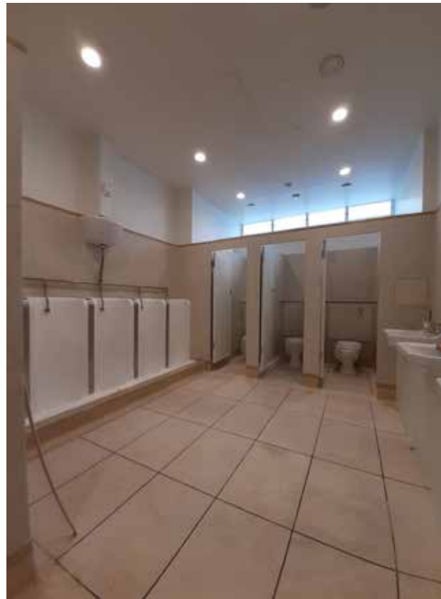
87 G.45 Men's Lavatory looking east
