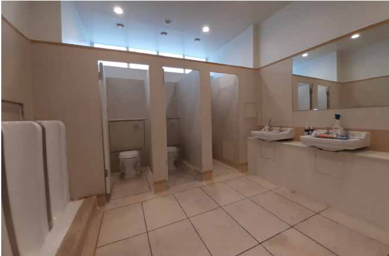
87A G.45 Men's Lavatory looking south
