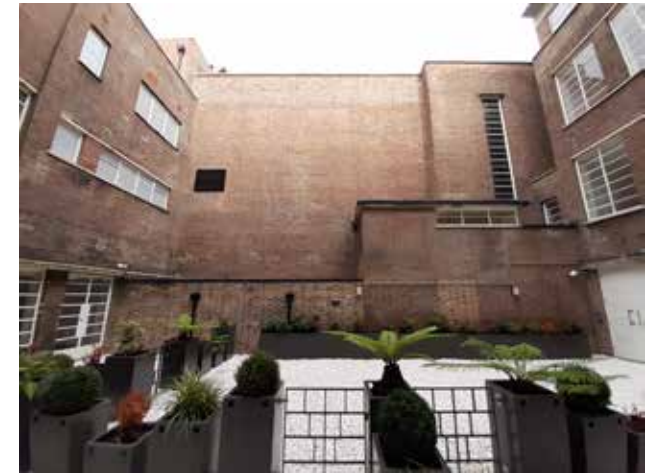
42 Service Court elevation looking north
