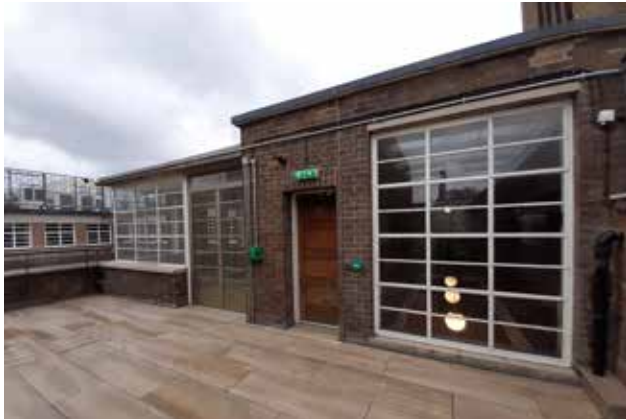
44 Flat roof over Assembly Hall Block
