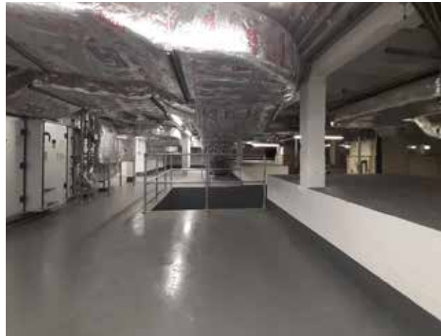
65 LG.43 Plant Room beneath Assembly Hall 1
