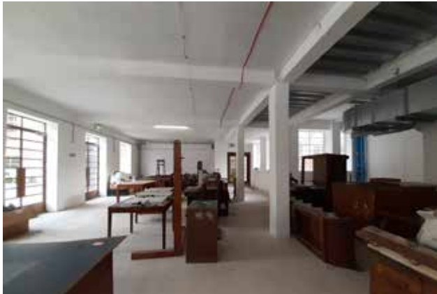
81B G.38 F&B Restaurant Cafe looking east to G.41 Entrance Hall
