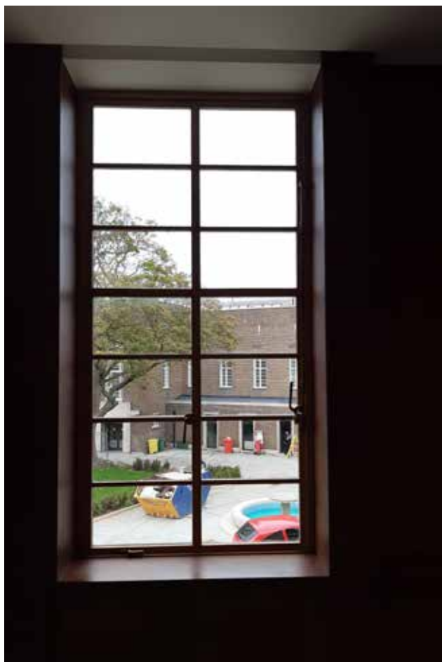
115A F.37 Member's Room, typical window to room
