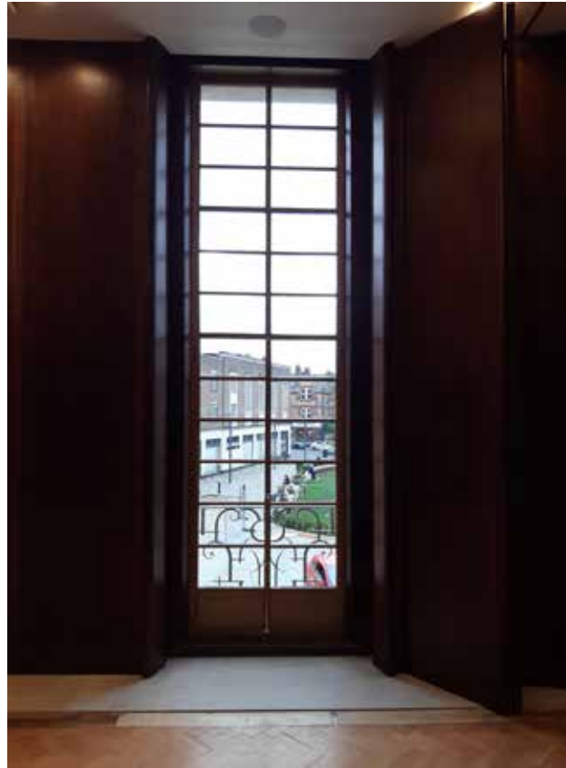
120B F.46 Committee Room, typical tall glazing to west elevation
