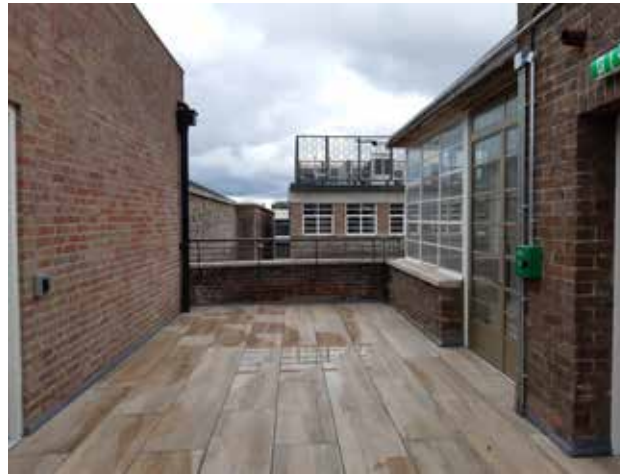
130A S.1a Roof Terrace looking east
