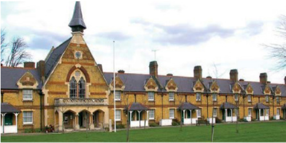
VIEW 1 - VIEW OF THE CENTRAL FORMER CHAPEL
