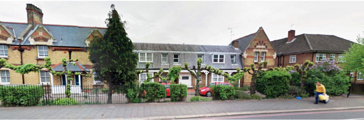
VIEW 2 - VIEW OF THE 1970'S INFILL BUILDING
