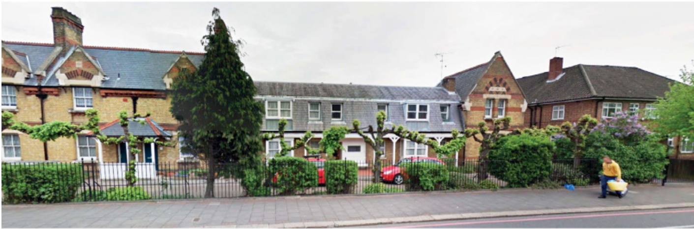
VIEW 2 - VIEW OF THE 1970'S INFILL BUILDING
