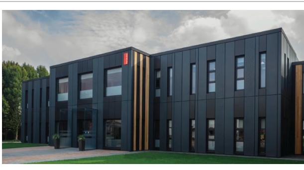
Figure 13 Modular building with external insulation and cladding.
