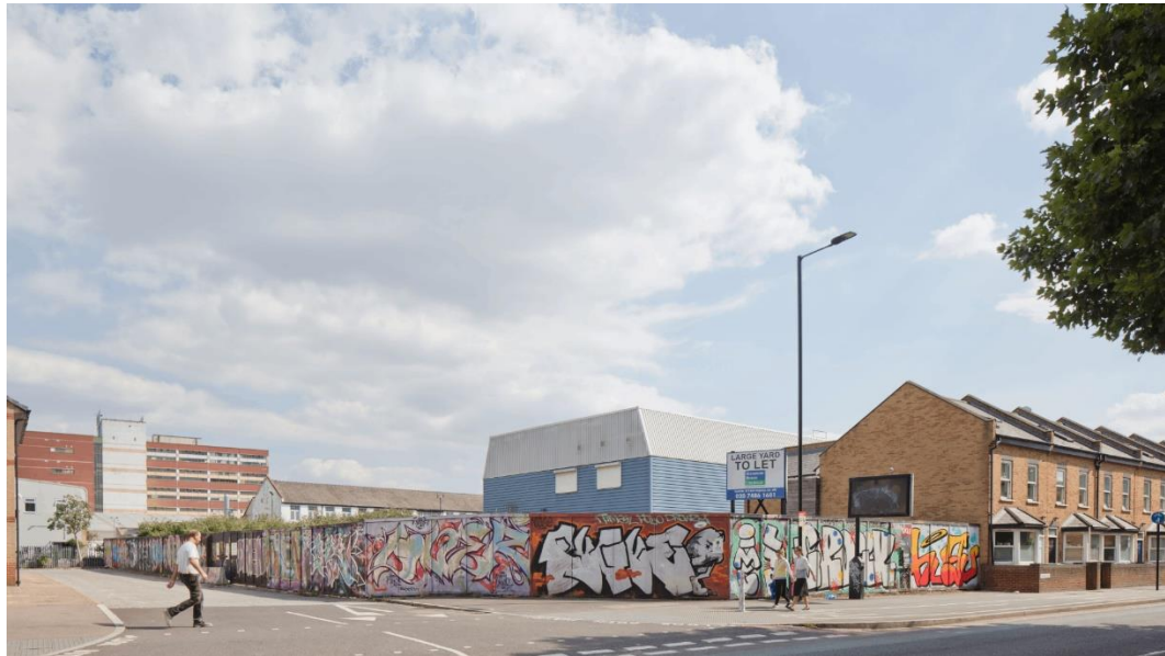
EXISTING SITE VIEWED FROM BROAD LANE
