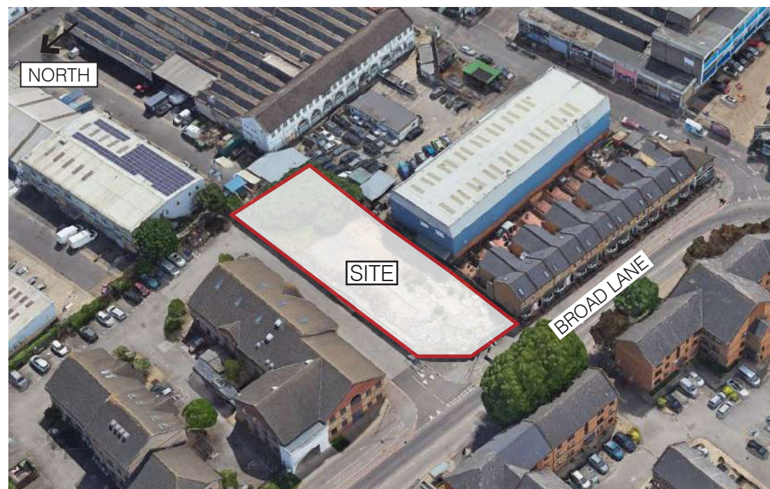
2. EXISTING AERIAL VIEW OF SITE
