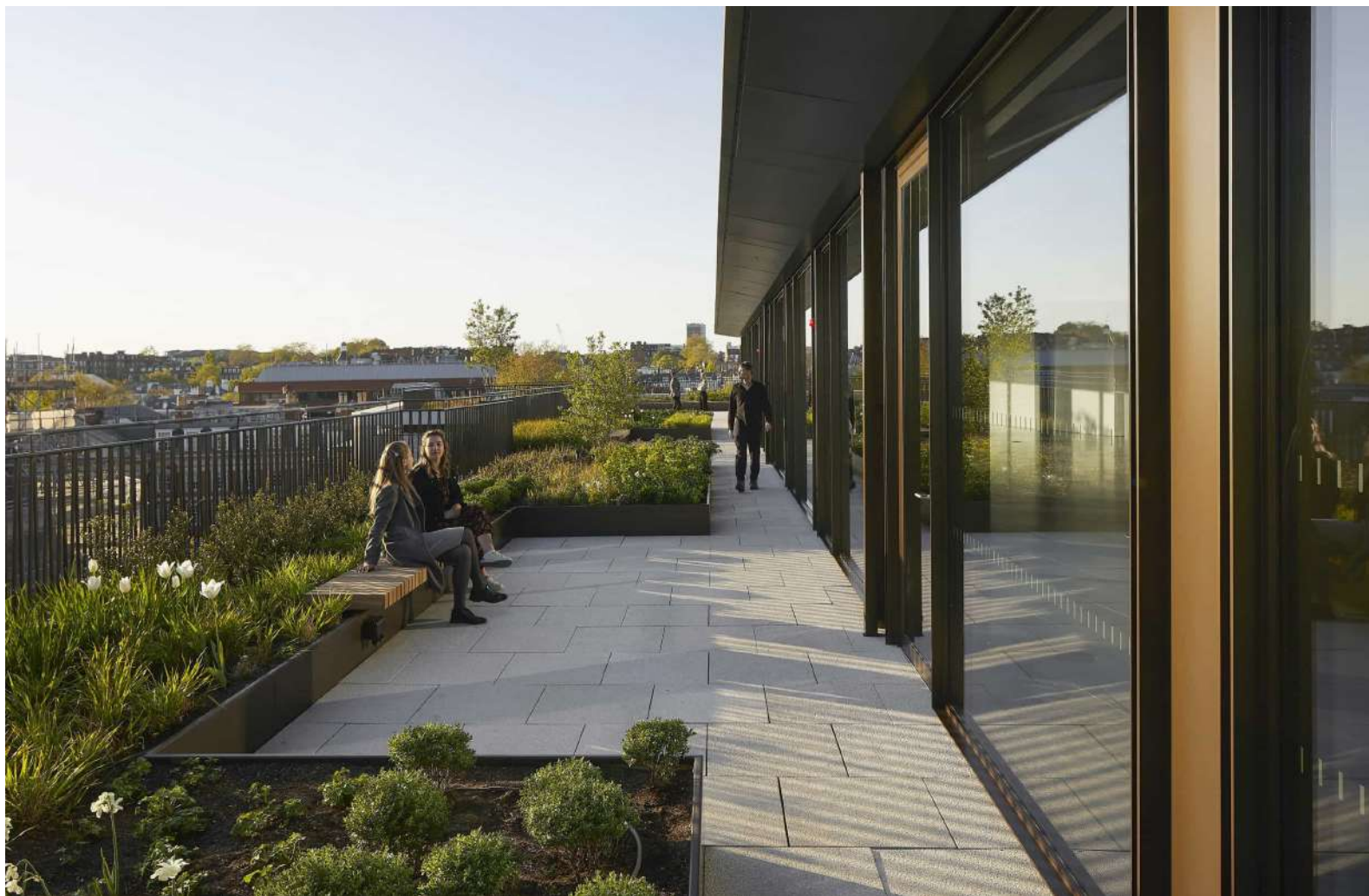
FIGURE 15 - EXAMPLE ROOF GARDEN (WRIGHT'S LANE, KENSINGTON)
