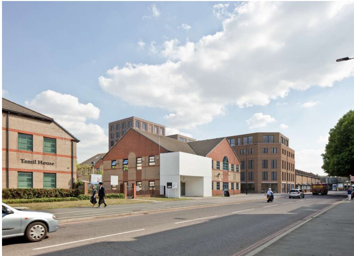
FIGURE 08 - PROPOSED BUILDING VIEWED FROM BROAD LANE NORTH OF SITE (BEFORE Q.R.P.)
