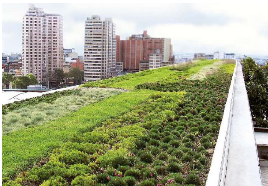
FIGURE 03 - EXTENSIVE GREEN ROOF BY ZINCO GREEN ROOF SYSTEMS
