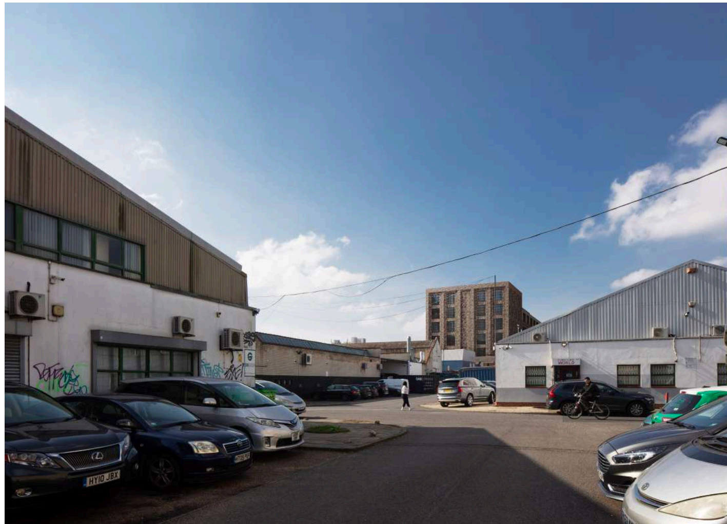
FIGURE 10 - PROPOSED BUILDING VIEWED FROM THE ARCHIVES AT HIGH CROSS CENTRE (BEFORE PRE-APP.)
