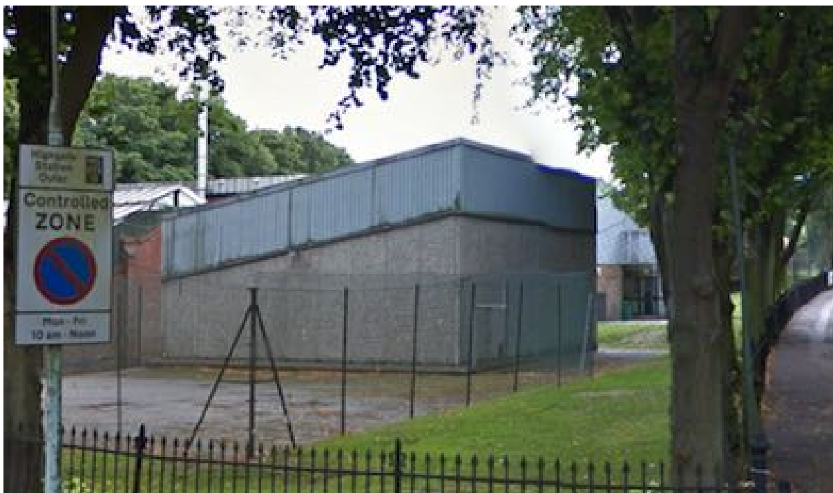
View of the northern Squash Courts building from the north, with hardcourt in front
