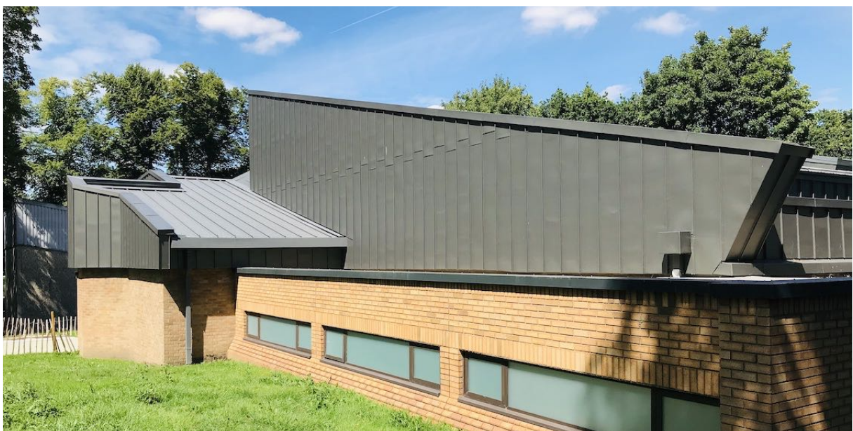
View of the MSC Pool Hall, refurbished in 2020 as part of a masterplan approach to the site
