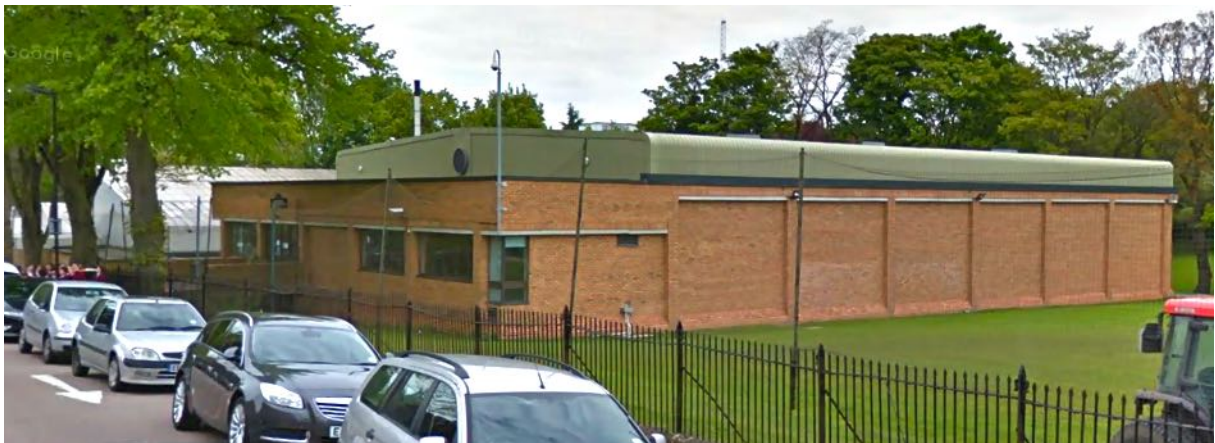
View of the MSC sports centre site from south, with the blank wall of sports hall to the MOL
