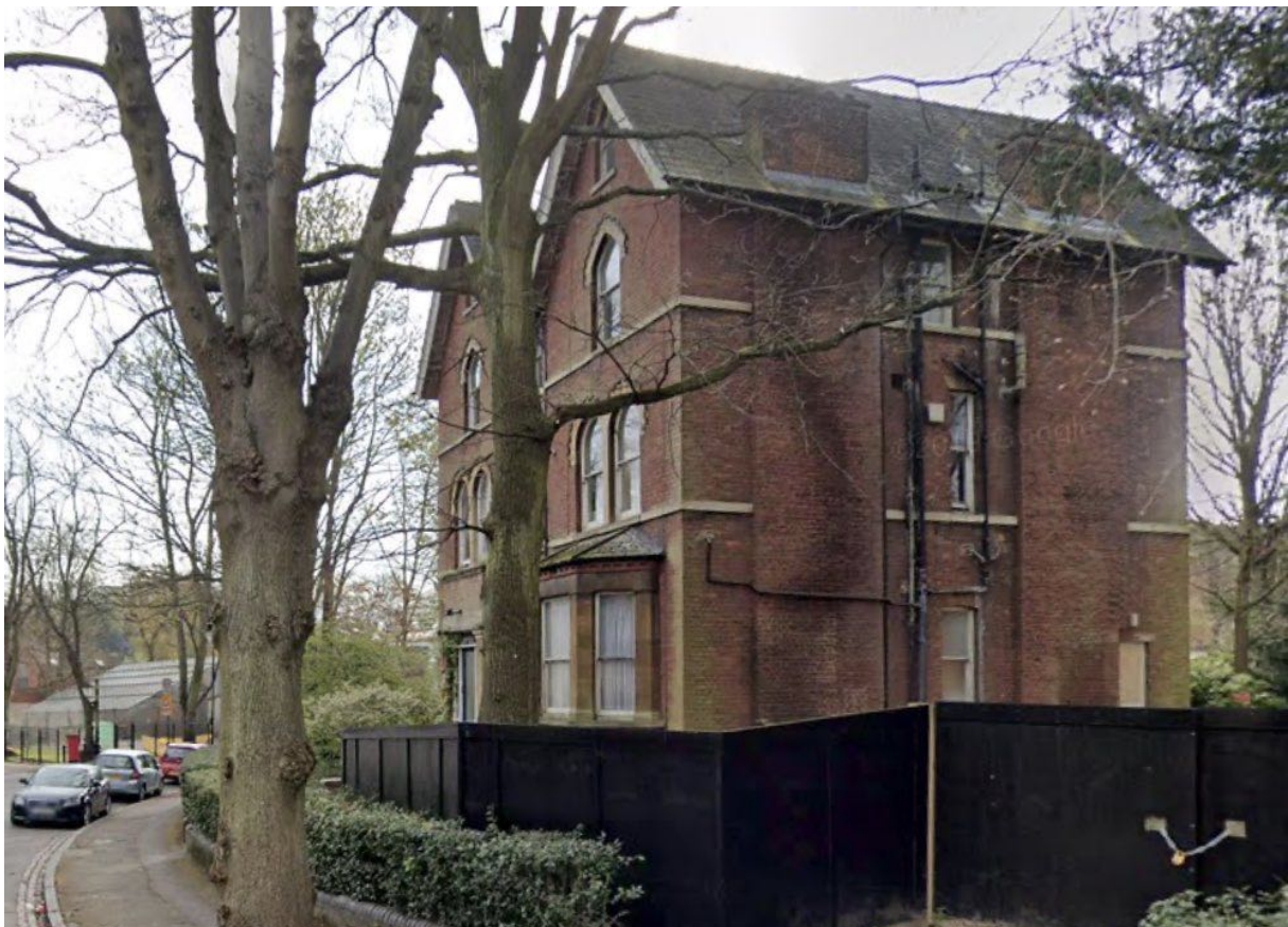
View of No.11 Bishopswood Road, example of Victorian villas in this locality
