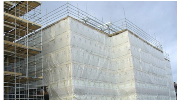
Monarflex Encapsulation Scaffold
