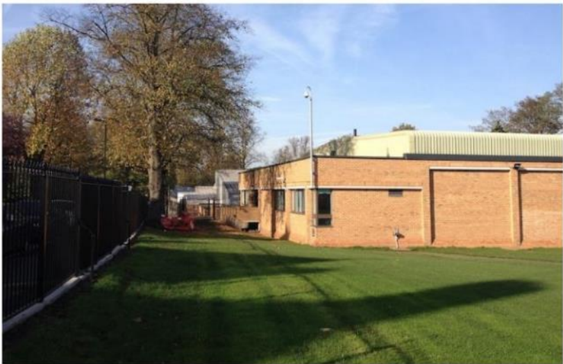
View of the MSC sports centre site from south, Bishopswood Road on the left behind railings
