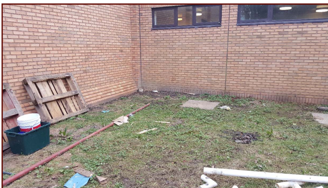
'Courtyard' area; sports hall on left and changing rooms on right (looking S)
