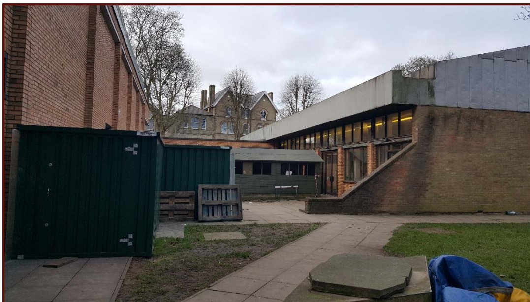
General view of 'courtyard' area (looking SW)
