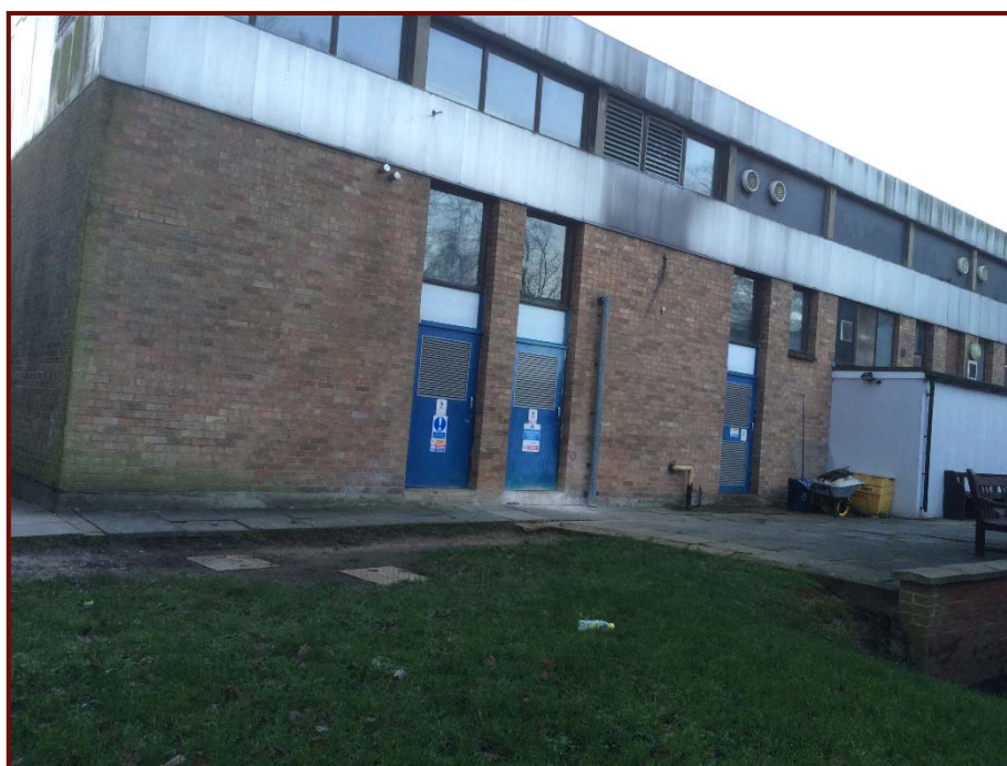
Swimming pool building showing plant rooms (looking S)
