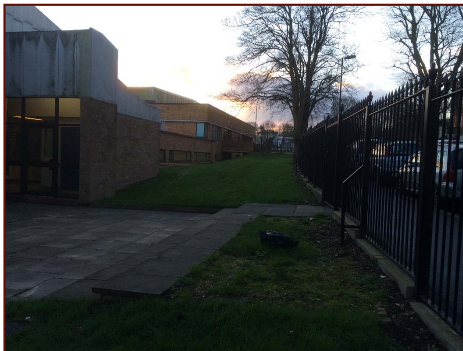
View along Bishopswood Road boundary (looking SE)
