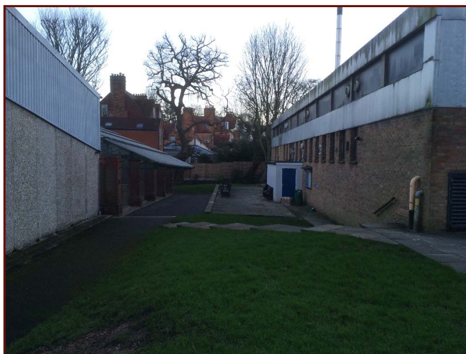
View along side of swimming pool boundary with games courts on left (looking NE)
