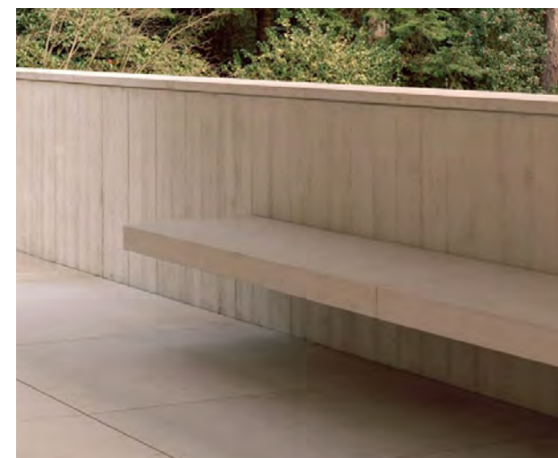
SEATS - FIVES COURTS Cantilever concrete seat
