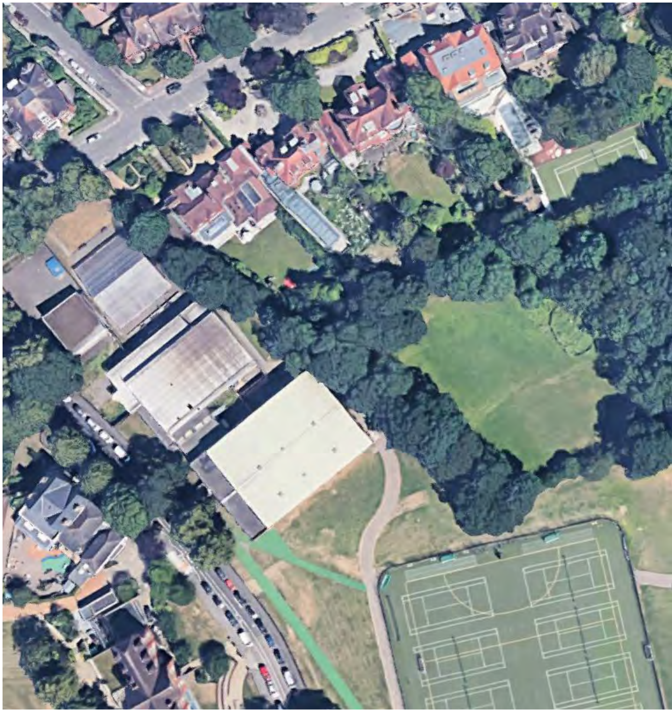
HIGHGATE MSC AERIAL VIEW
