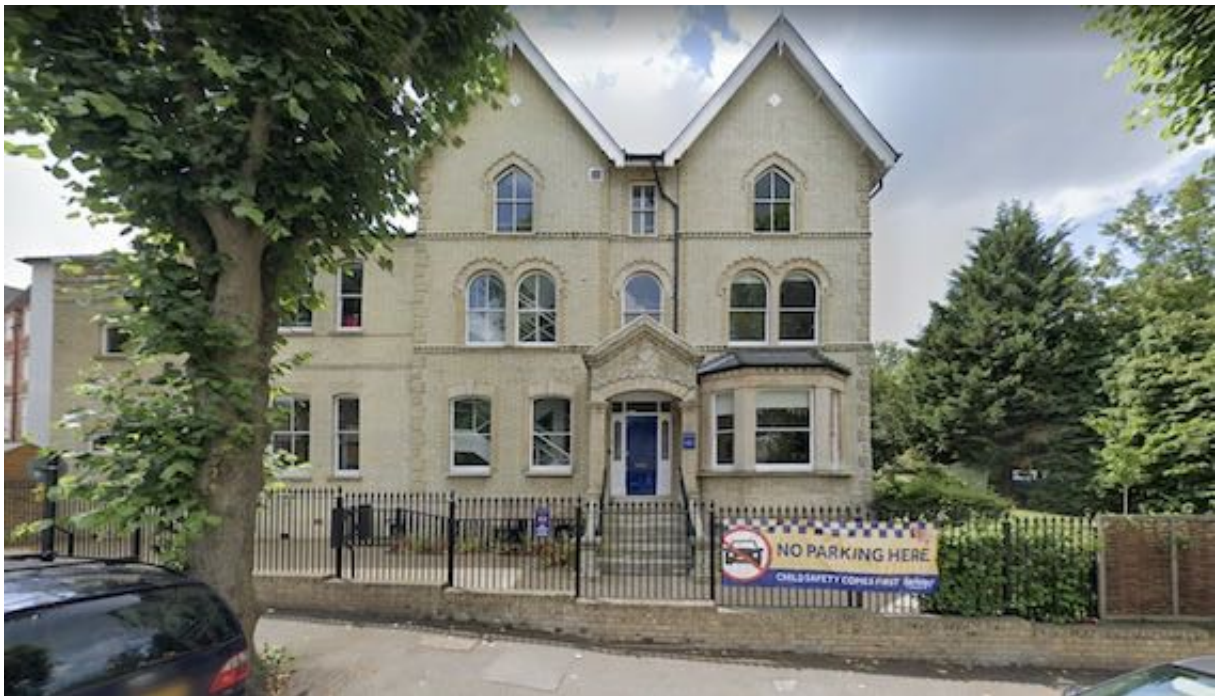
View of Grindall House opposite from existing MSC entrance
