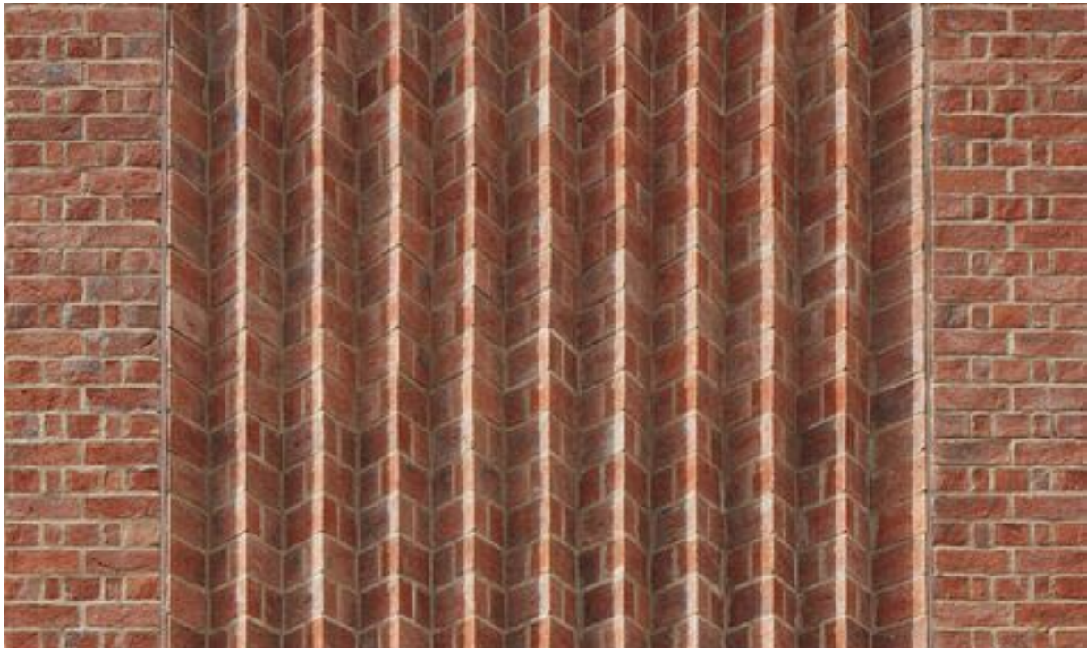
Example of brick detailing in the west elevation bays, with rotated bricks
