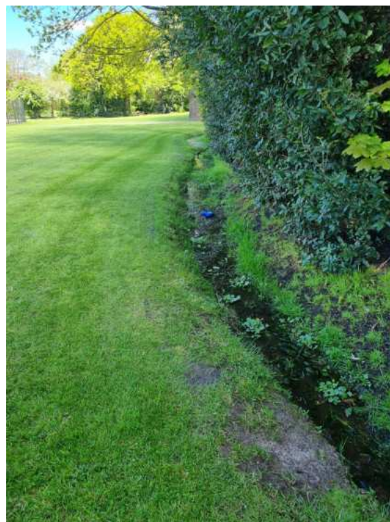
Figure 2.3: Existing swale to the east of the sports pitches requiring clearance and improvements to increase capacity.
