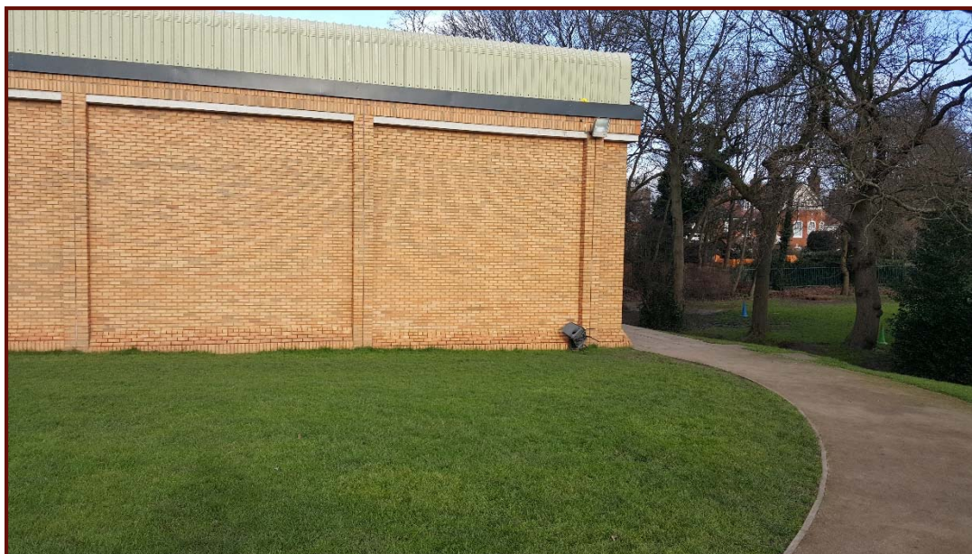
View of SE elevation of sports hall (looking N)
