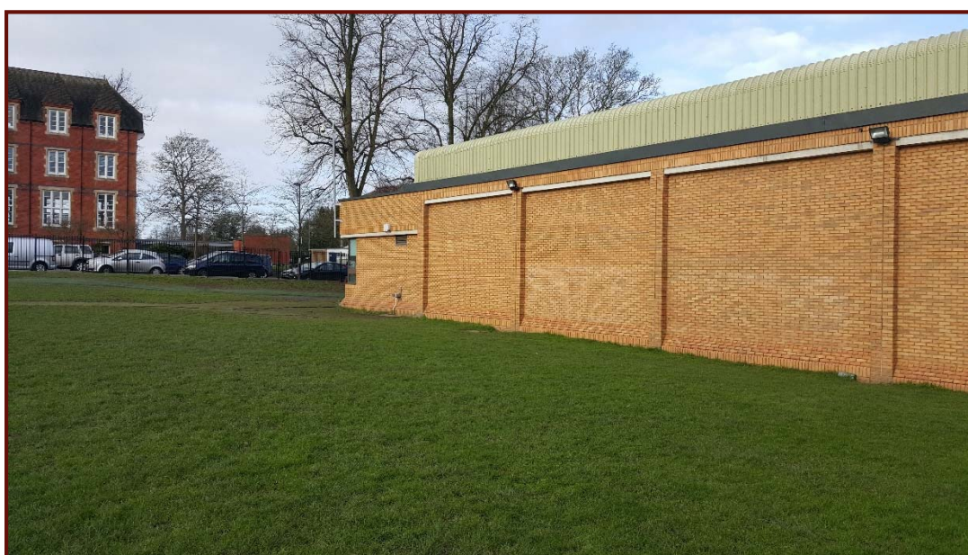
View of SE elevation of sports hall (looking NW)
