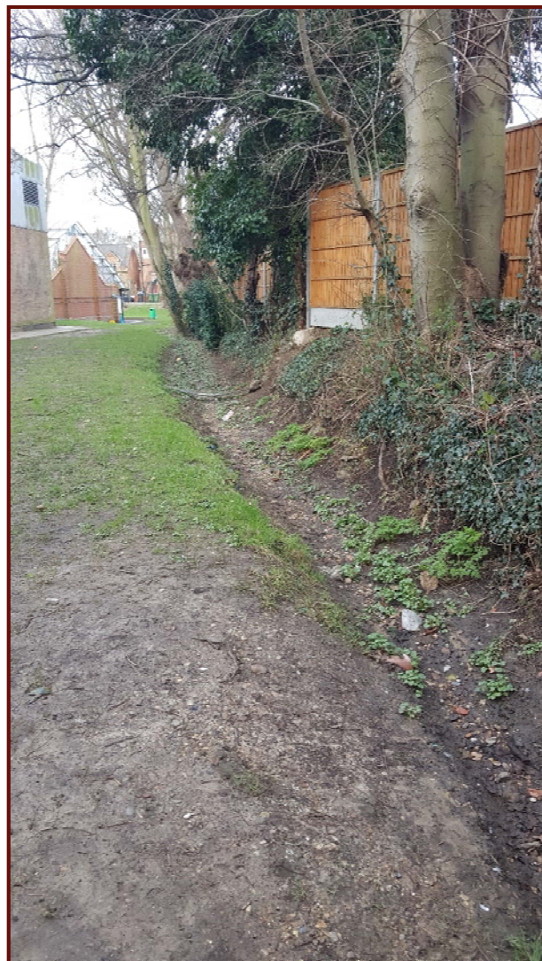
Shallow tree-lined drainage ditch to NE of swimming pool (looking NW)
