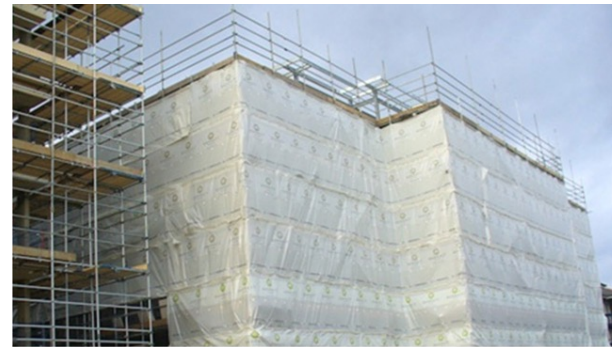
Monarflex Encapsulation Scaffold
