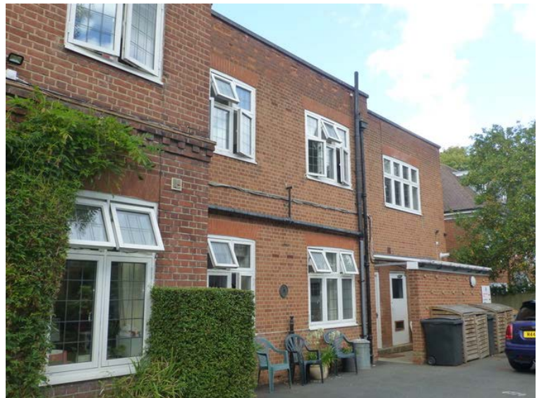
Figure 7: The eastern extension on View Road
