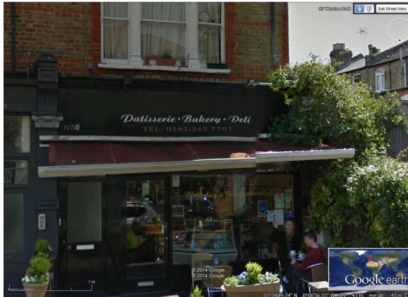
The new canopy
