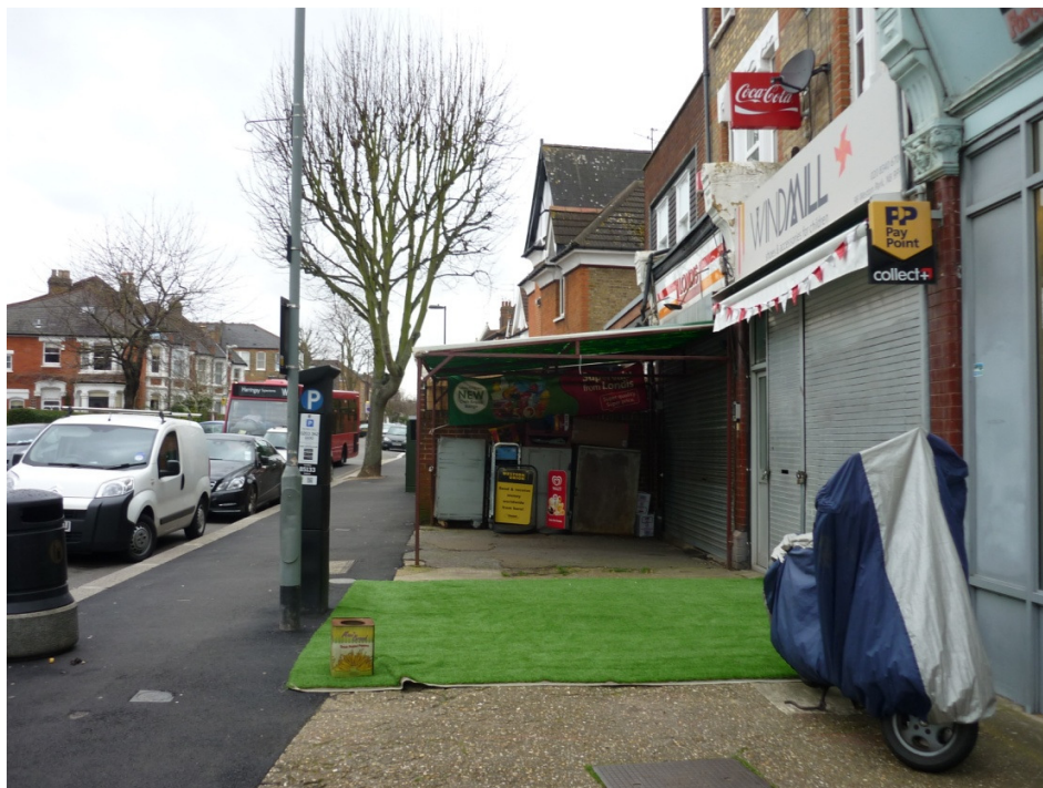
3) Canopy on buildings opposite
