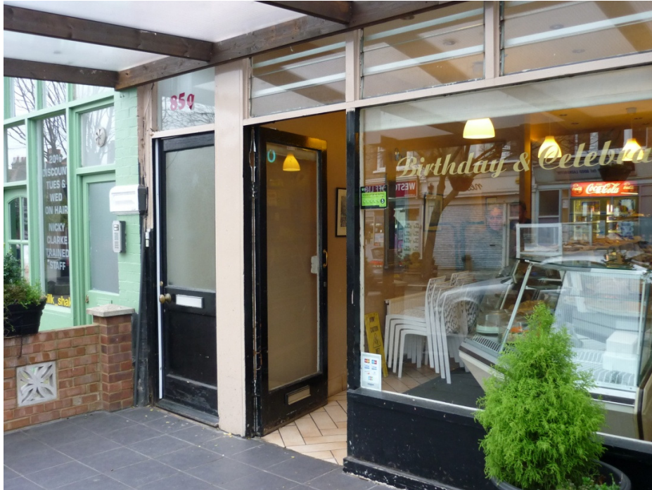
2) The Taken down canopy from inside.
