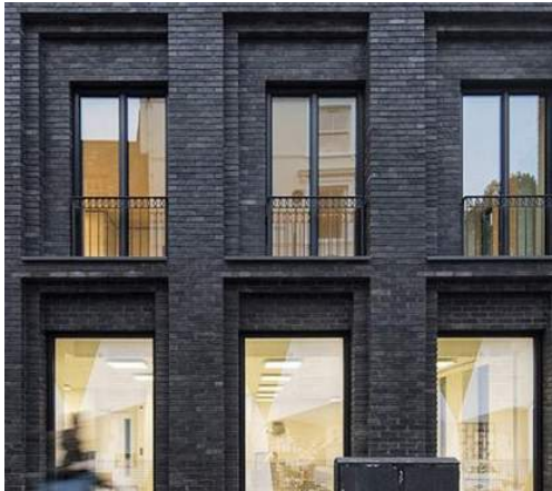
Brickwork (Recess Detail)
