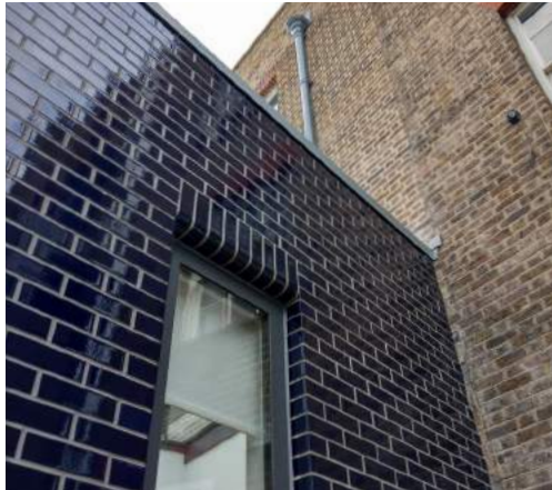
Brickwork (Blue Glazed)
