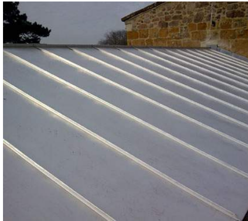
Standing Seam Roof
