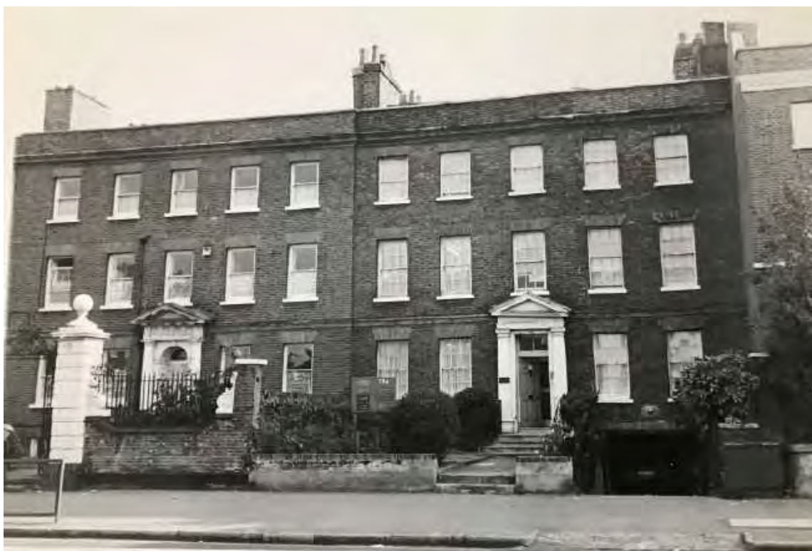
Figure 23 – Nos. 794-796 (thought to be c.1977 due to windows boarded on No.792)
