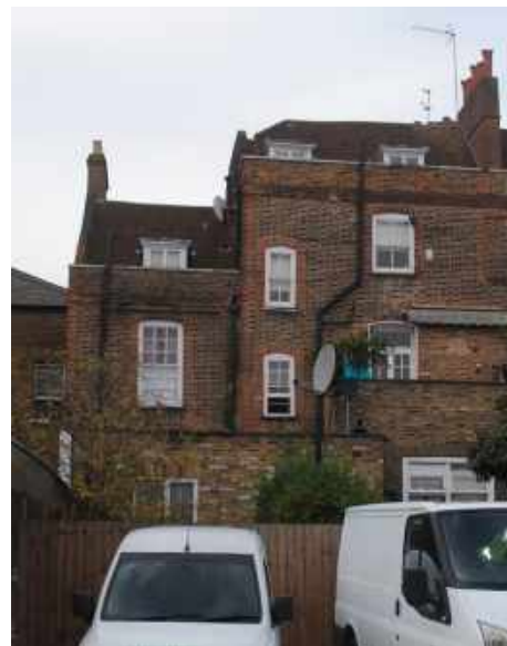
Figure 54: Rear of No 808 High Road - 2017
