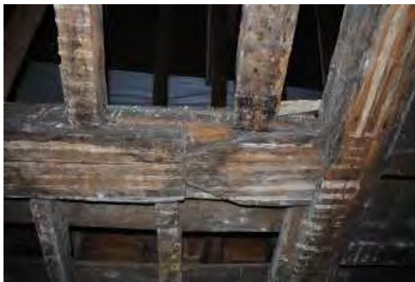
Figure 33 – Reused bridging beam with dovetail joint found in the roof of Percy House
