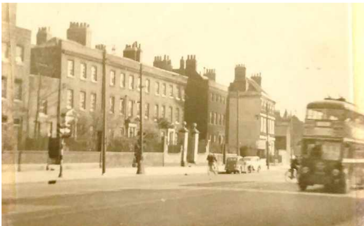
Figure 17 - May 1939 of 790-800 High Road – note that the boundary walls of No. 794-803 are all the same height as No. 796 (Percy House) and Nos. 794 and 798 are symmetrical, each side of Percy House.
