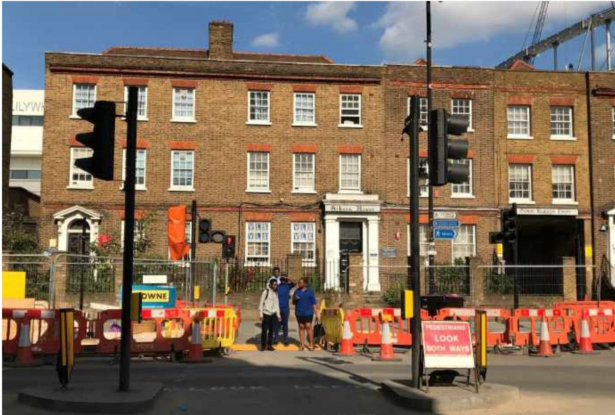
Figure 42: Nos. 802 (left) and 800/ Gibson House (right) - 2017
