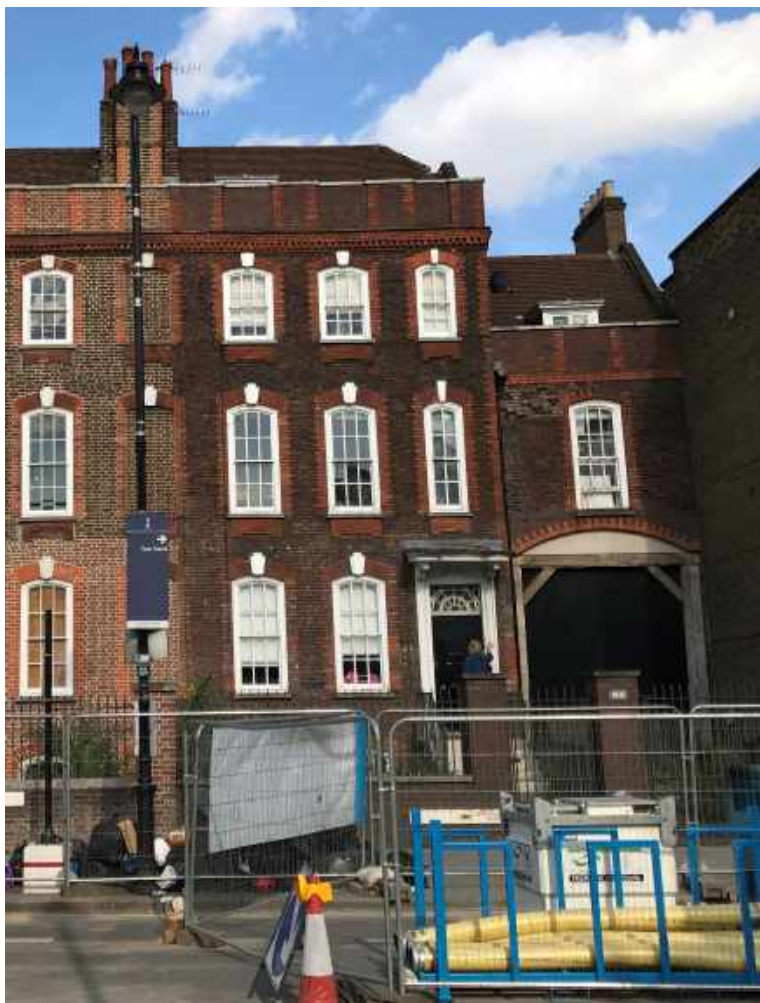
Figure 55: No 808 High Road - 2017
