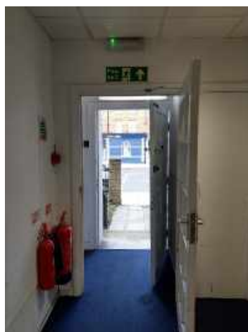
Ground Floor Hall and Stair – No. 802
