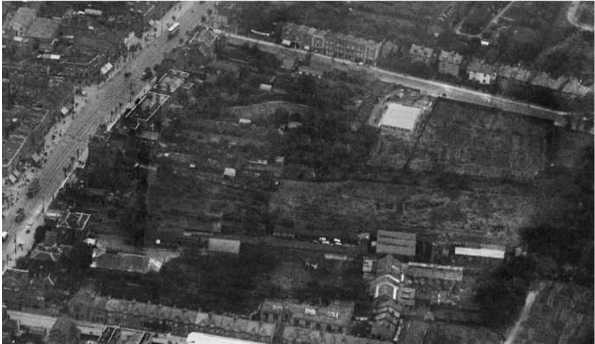
Figure 60: An oblique aerial photo of 1923, from the south showing the rear gardens of Northumberland Terrace.
