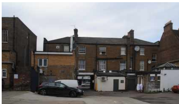
Figure 50: Nos. 804-806 High Road – Rear elevation 2017.
