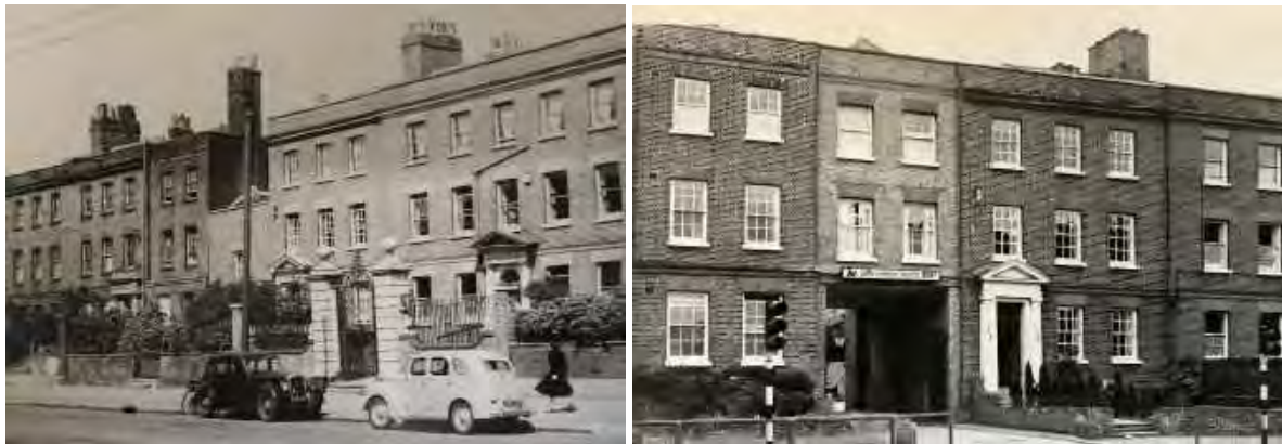
Figure 36: No.798 High Road in 1950 (left) and 1980 (right) showing change of ownership boundary, boundary treatments and the demolition of the two storey extension to make way for vehicular access route.
