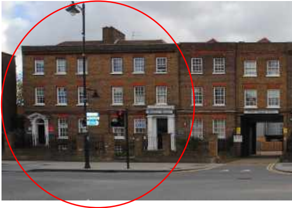
Figure 29 – Northern Block (Nos. 802 – 800)
