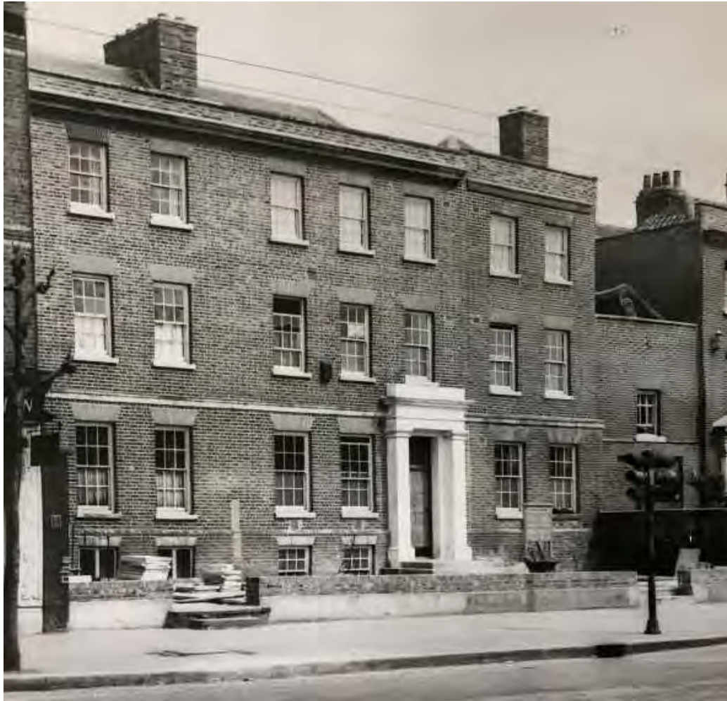
Figure 24 - 798-802 – c.1960 showing 800-802 under refurbishment, prior to No.798 2 storey extension being sold to No.800 and demolished to provide a raised bridge over the car access.
