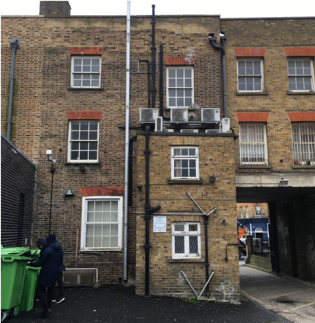
No. 798 High Road - existing rear elevation
