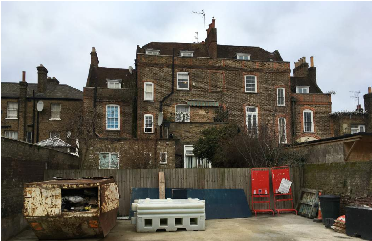
No. 808 High Road - existing rear elevation
