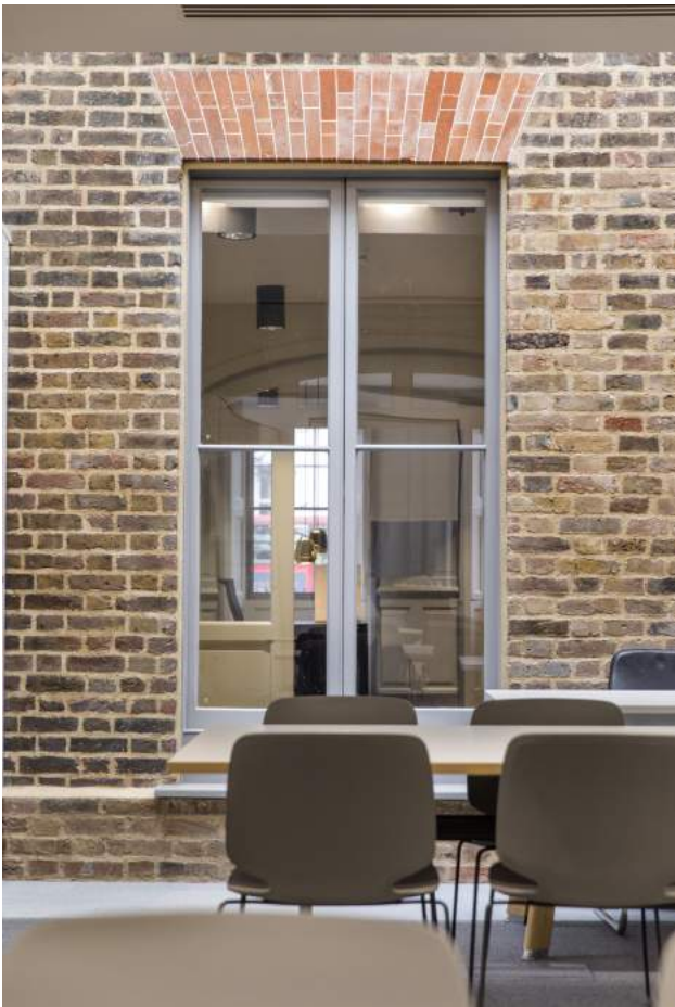
Percy House, framing of the rear elevation
