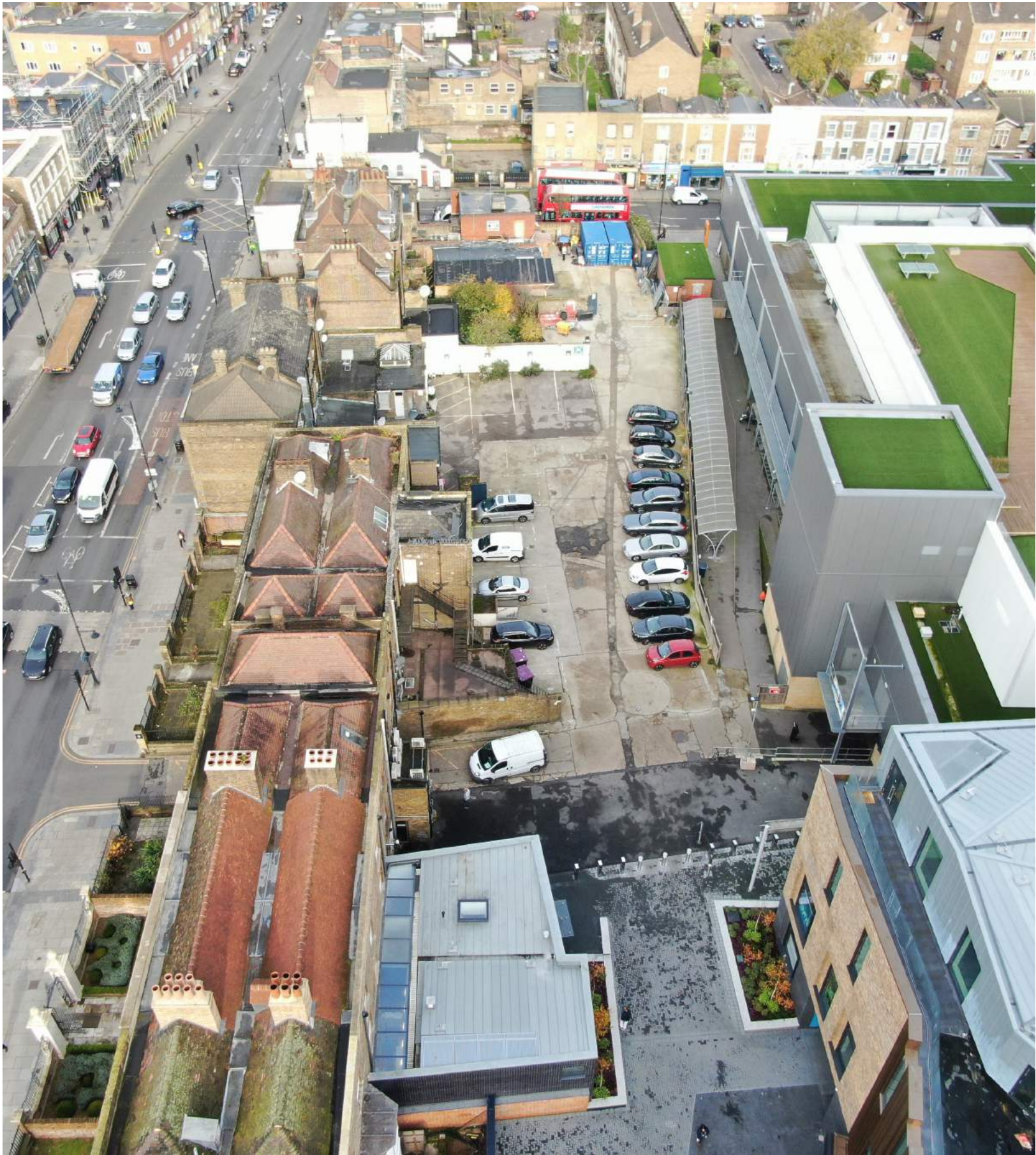
Site aerial view
