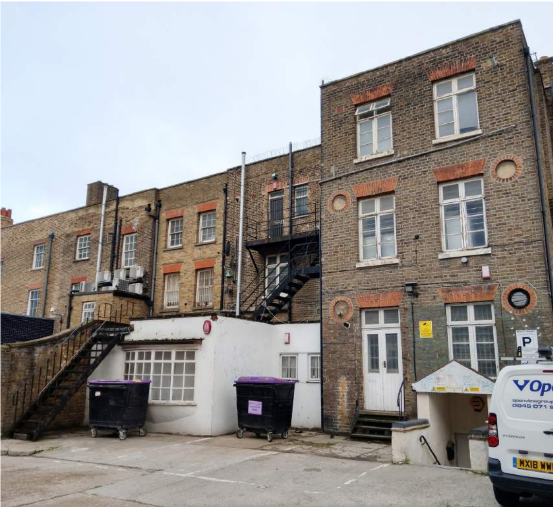
No. 800 High Road - existing rear elevation
