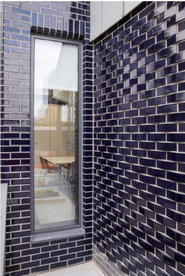
Percy House, brickwork detail to rear extension
