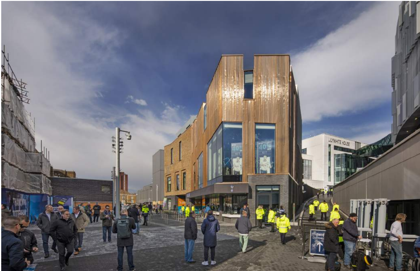
Paxton Development (Phase 1) - looking north through Paxton Place
