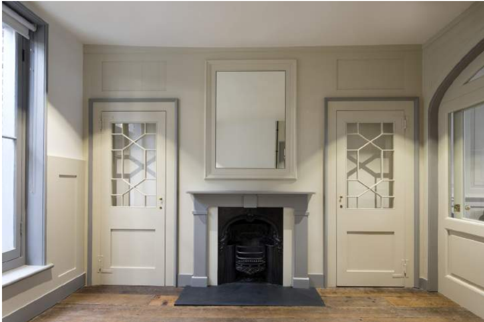
Percy House Restoration as the TH Foundation - ground floor interior
