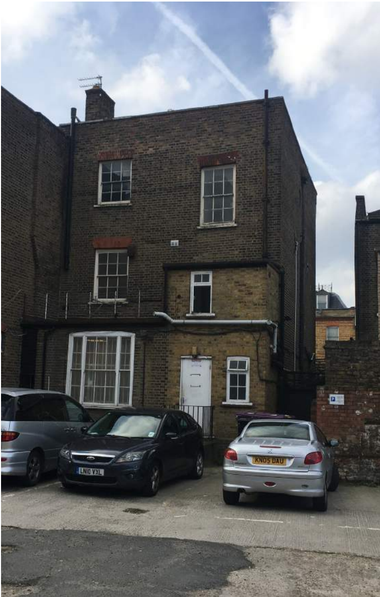
No. 802 High Road - existing rear elevation
