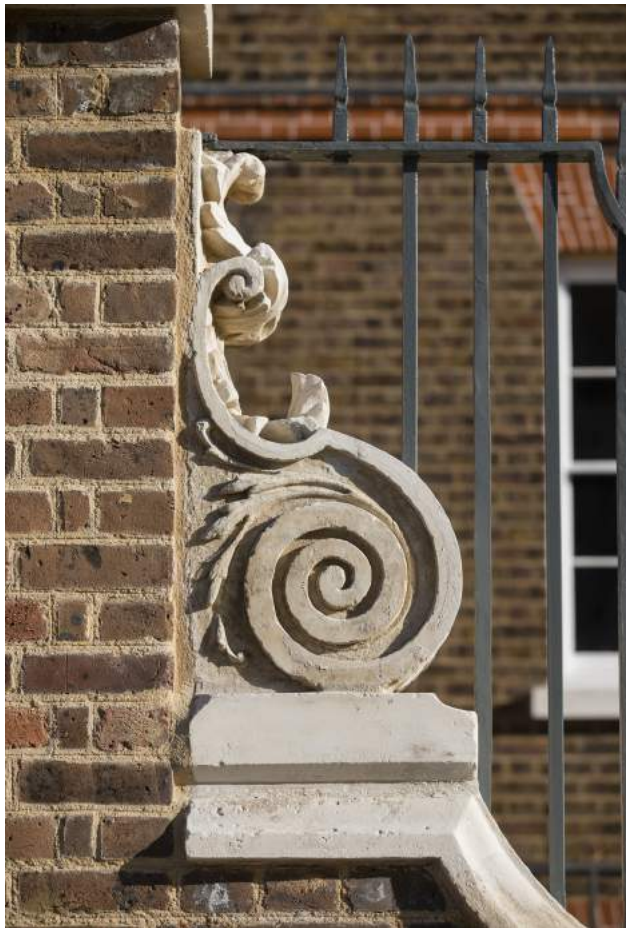
Percy House, No. 796 High Road - restored gate detail
