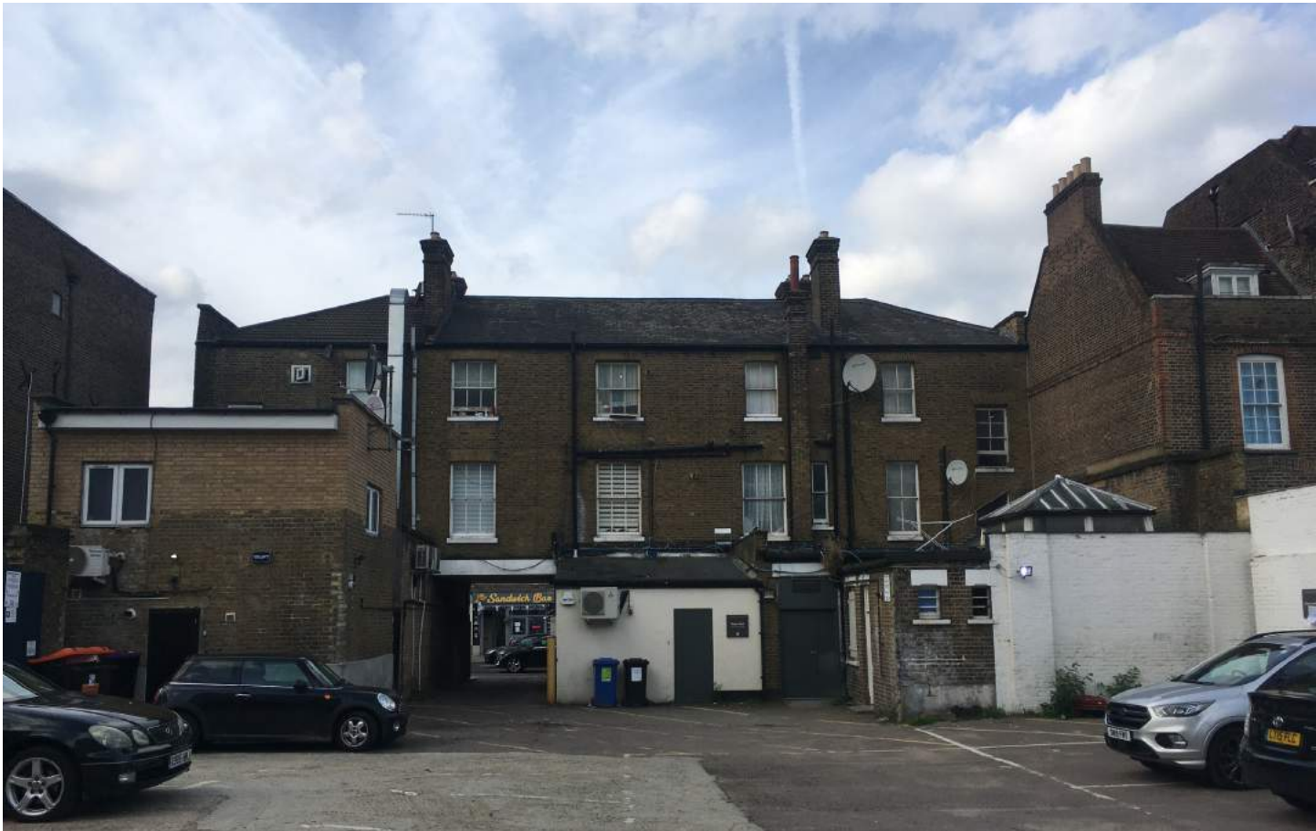
No. 804-806 High Road - existing rear elevation
