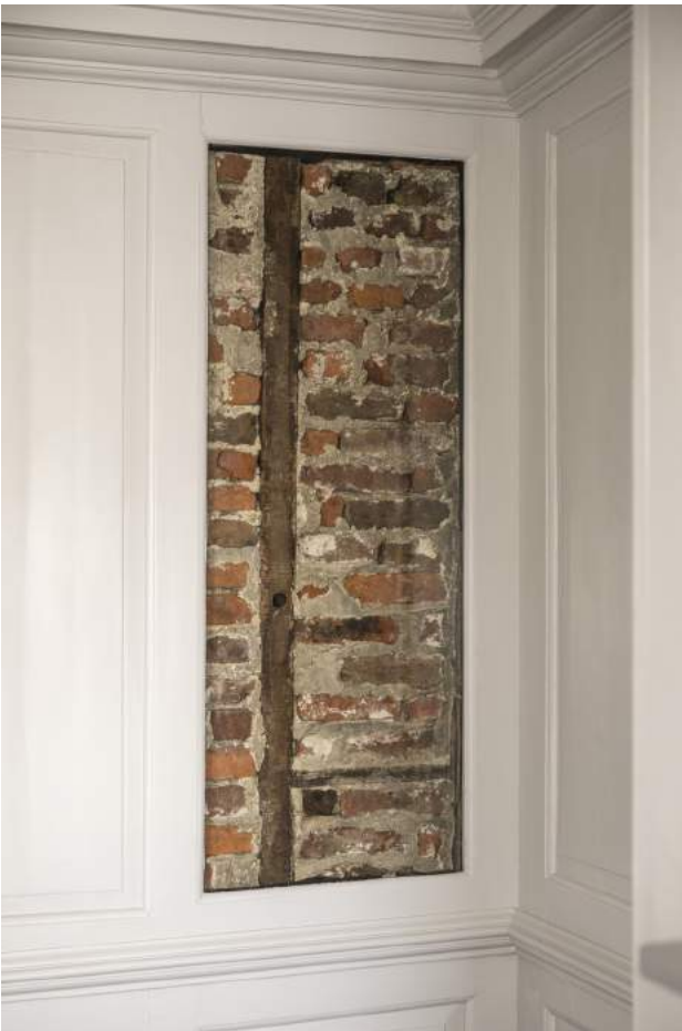
Percy House Restoration as TH Foundation - interpretation
