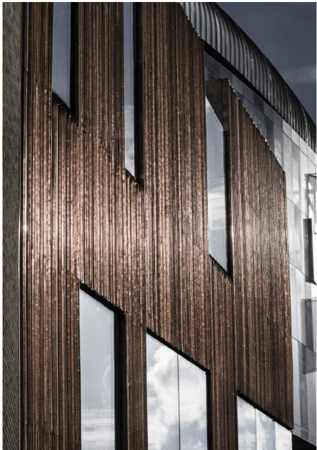
The Paxton Building - completed bronze cladding
