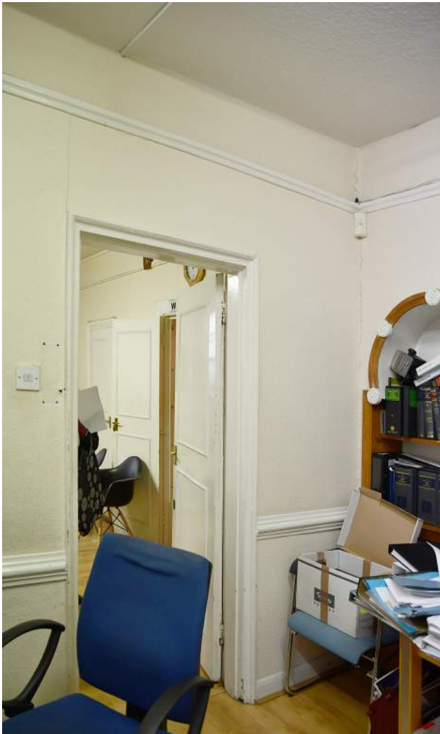
No. 800 High Road - typical first floor interior
