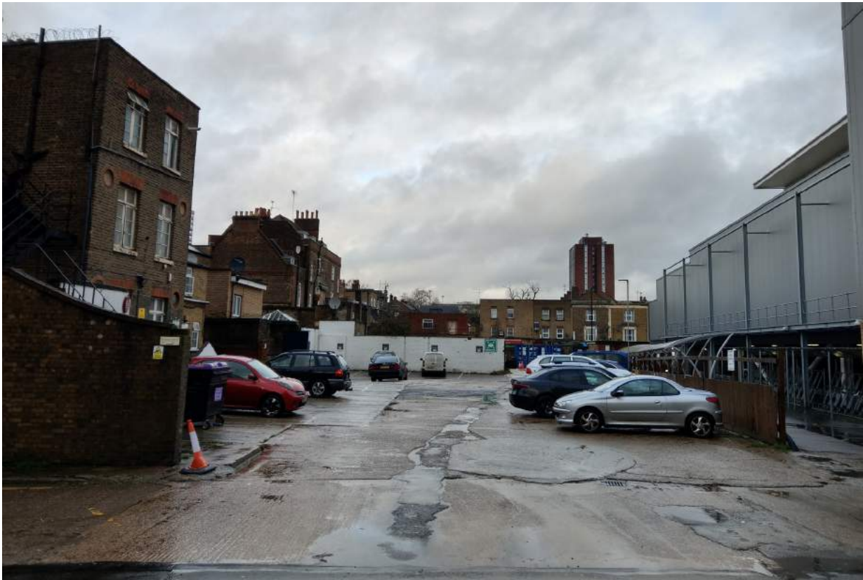
Site looking north from Paxton place
