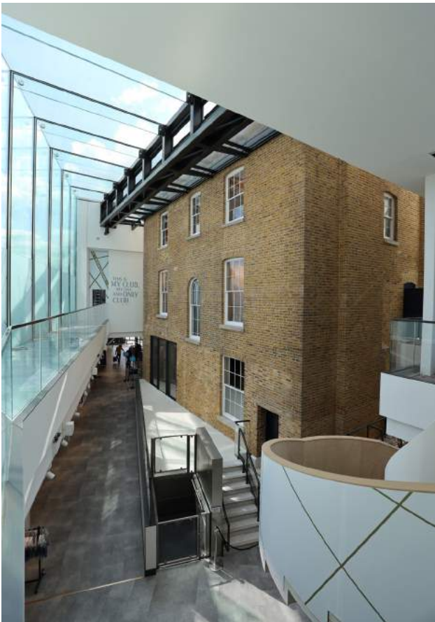
Warming House, restored as part of the NDP
