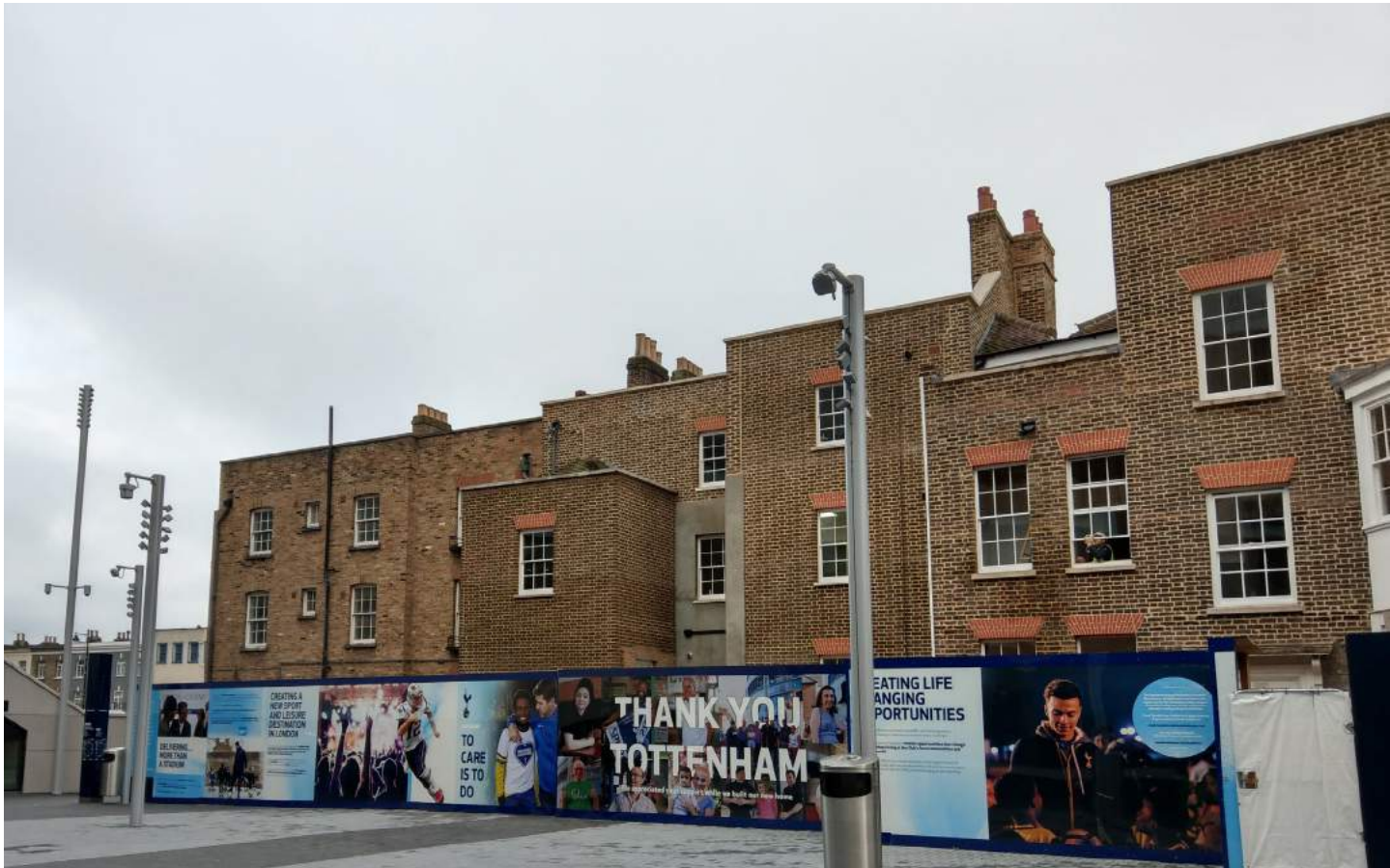
Paxton Development (Phase 2) - restored rear elevations of Nos. 790 to 794 High Road
