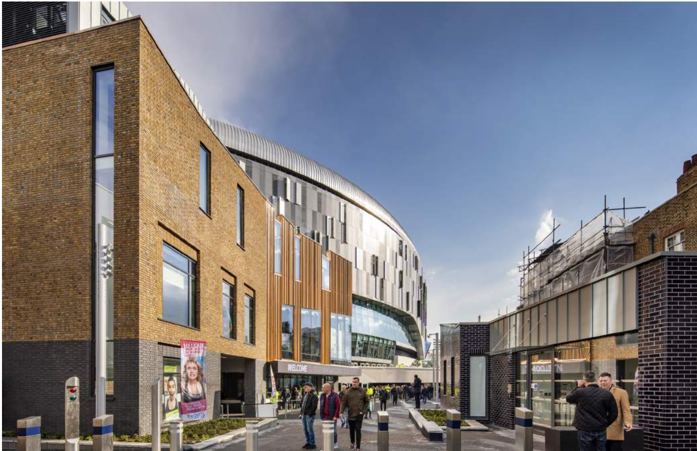
Paxton Development (Phase 1) - looking south through Paxton Place
