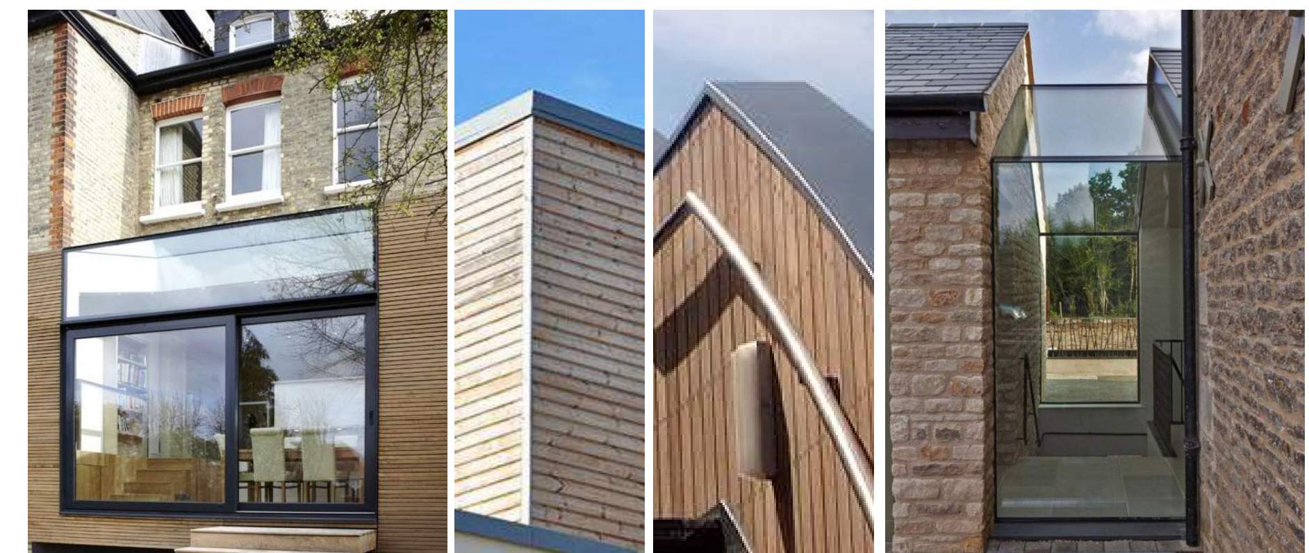
Dark grey metal window frames Metal coping Glazed element between old & new
