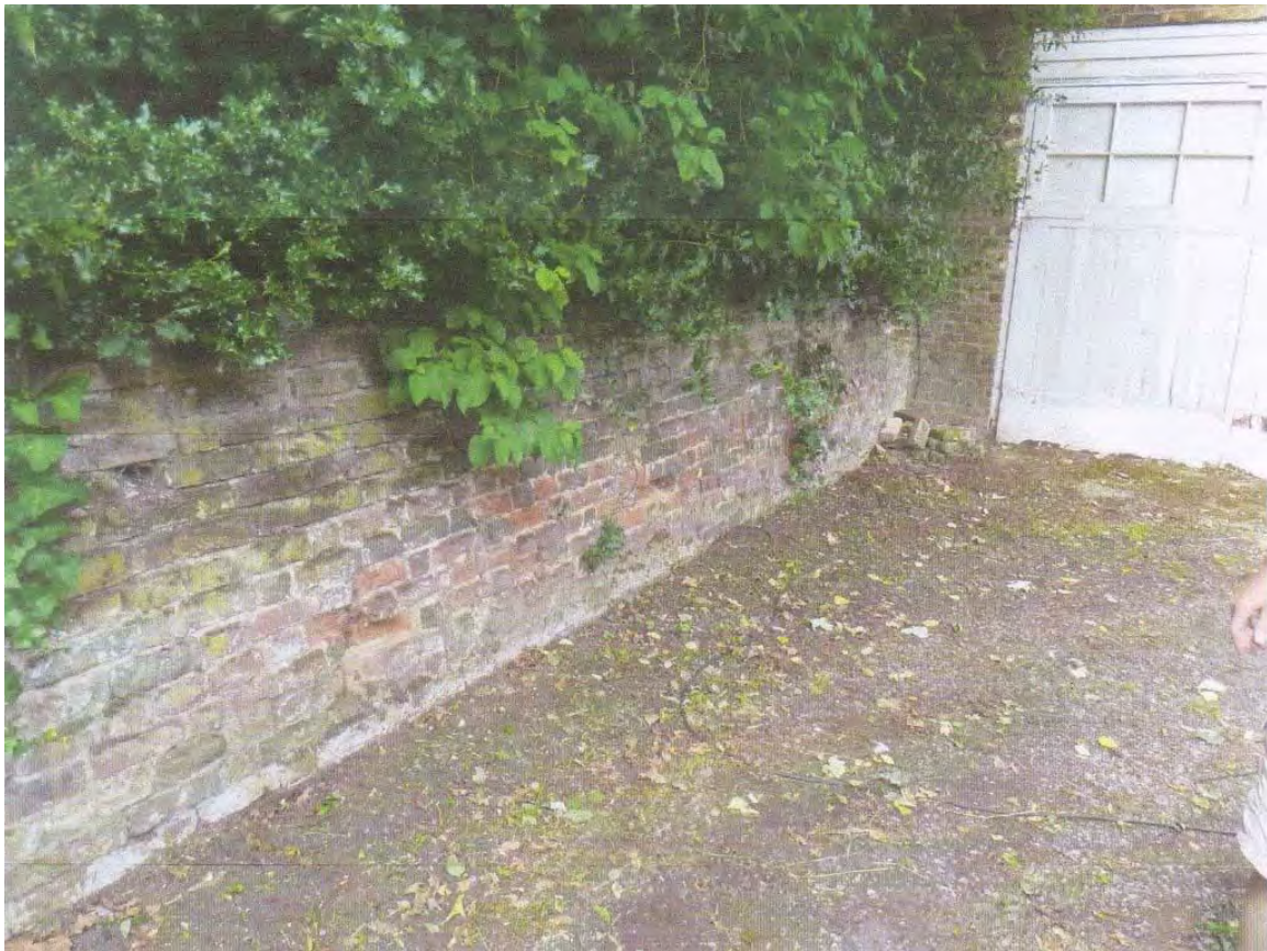
Figure 3: Boundary wall at the Coach House. Section of the old wall (note old red brick laid in lime mortar) running to junction with the Coach House. The old wall has been cut back and the Coach House built up to the wall so that the far sides align. The Coach House is Victorian yellow stock brick.
