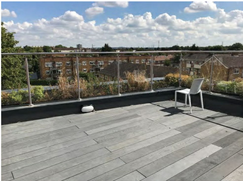
Photo 6: Communal Roof Terrace, fronting onto Chesnut Road
