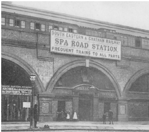
Typical London Railway Arches
